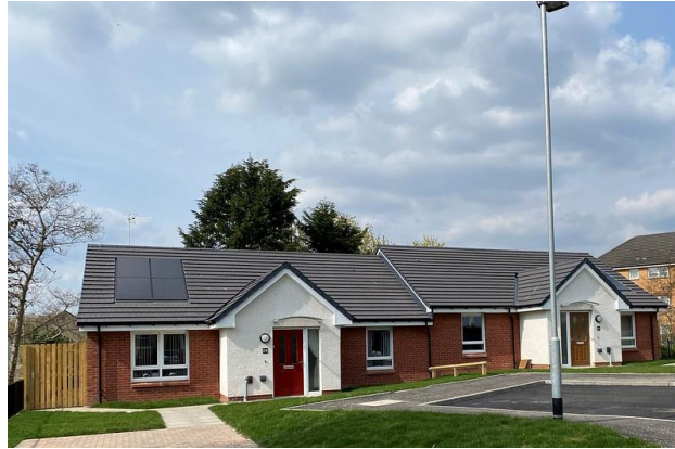
Caledonian Avenue/Nobles View, Bellshill North Lanarkshire Council
