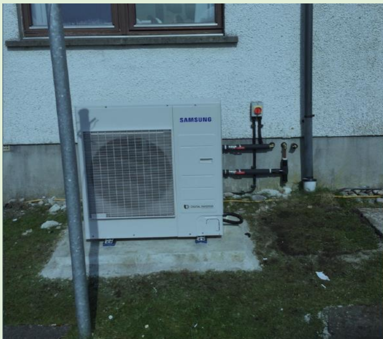
Image of an air source heat pump on a HHP home in the Outer Hebrides
