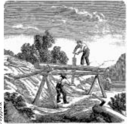
Sawing logs by hand using a large pit-saw.
