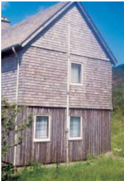
1970's social housing at Kyle of Lochalsh uses preservative treated western red cedar shingles.
