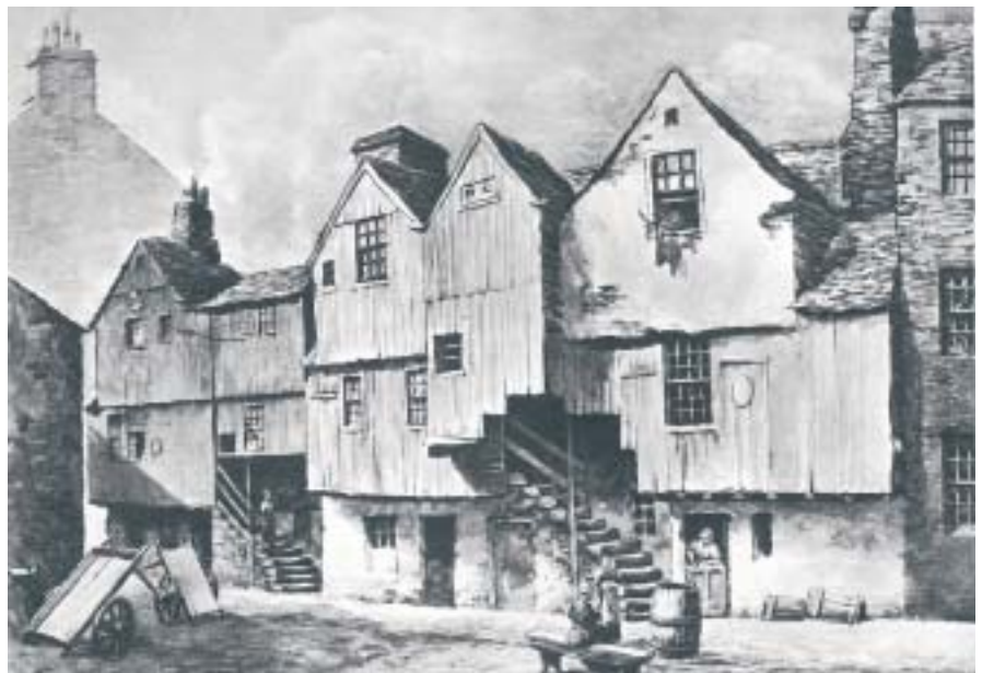
Wooden gallery on a house at 77 Saltmarket, Glasgow.
