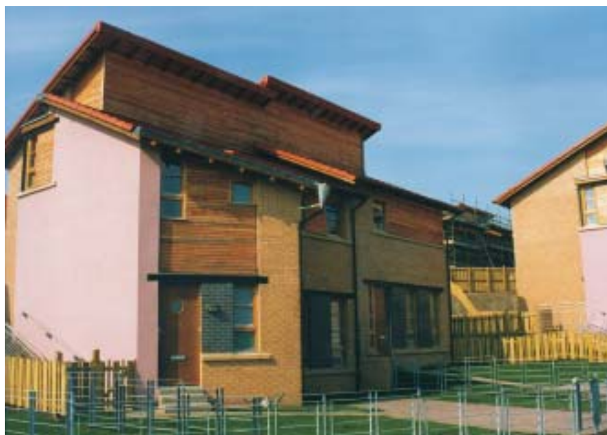
Whinhill Housing, Greenock by Chris Stewart Architects.
