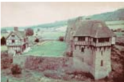
ABOVE Stokesey Castle's wooden defences are raised to the top of the wall in the form of hoards, and give some idea of what 14th century Scottish fortified houses might have looked like.
