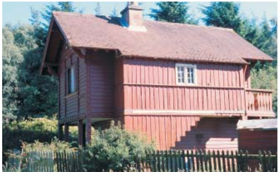
Swiss Cottage, Fochabers, c1820 was built to the pattern book designs of John Claudius Loudon and is one of the oldest surviving timber-clad buildings in Scotland.
