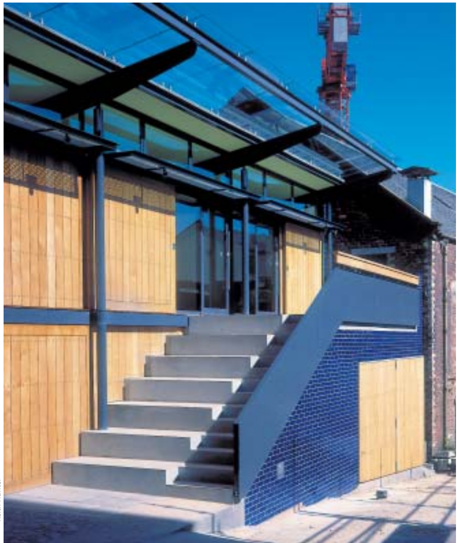
Scottish Poetry Library by Malcolm Fraser Architects uses uncoated European oak in its sliding screens and doors.
