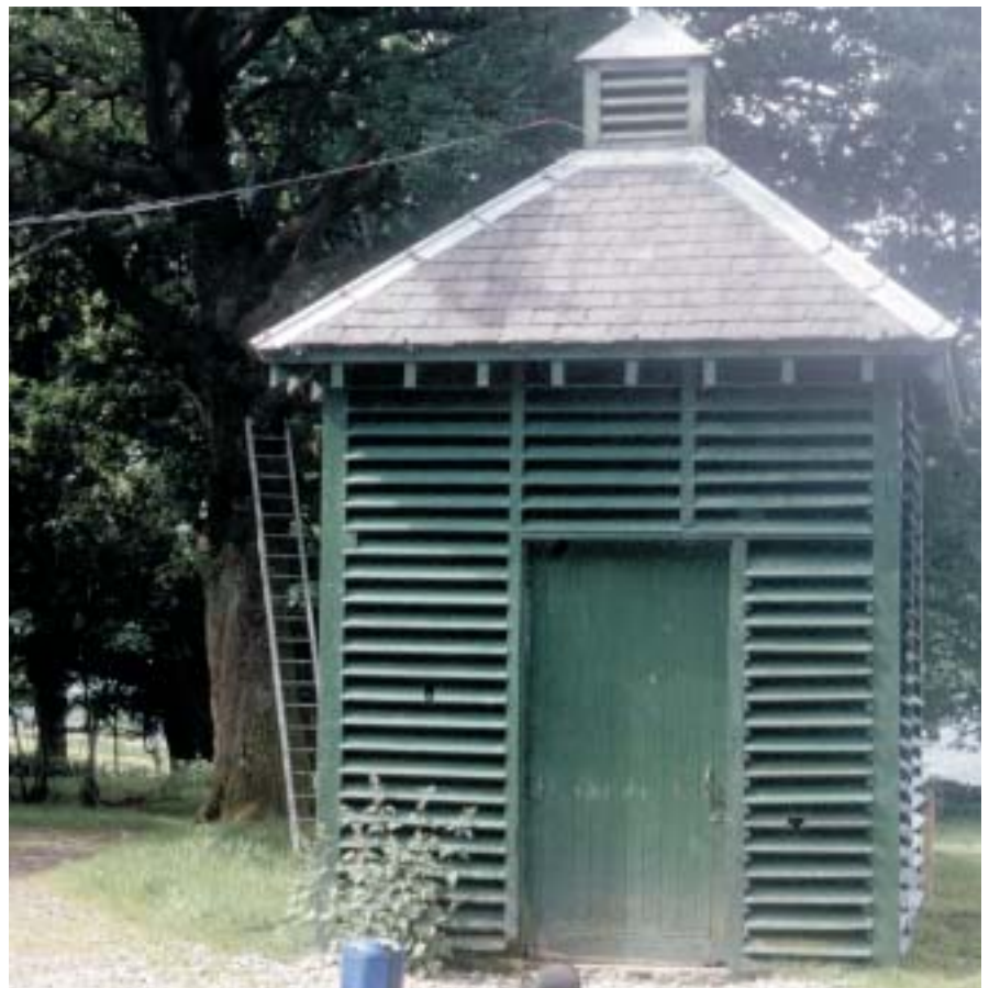
A late 19th century deer larder at Loch Hourn, one of the wettest places in Scotland. Well-designed and well-maintained timber cladding is suitable for our most maritime climates.
