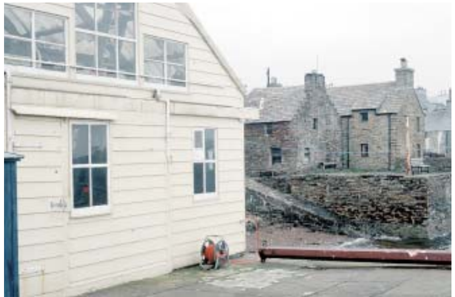
Late 19th century timber-clad fisherman's store in Stromness, Orkney has been painted a light, bright colour, a more traditional finish in Scotland than dark colours.
