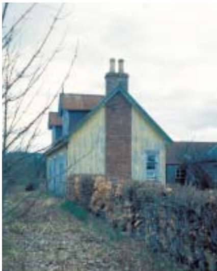
These brightly painted pre-fabricated houses were erected in many parts of the Highlands in the mid to late 19th century.
