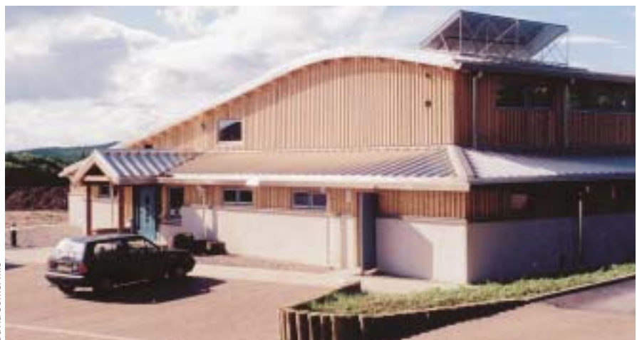
BELOW Locally-grown western red cedar cladding was used on the Ardross Millennium Project, near Alness by David Somerville Architect.
