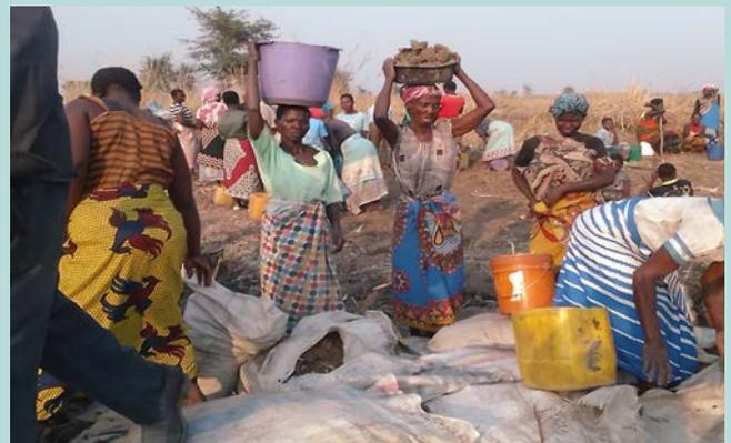
Figure 26: Community members filling up the polypack sacks with soil as they rehabilitate the waterway. Image by Alex James
