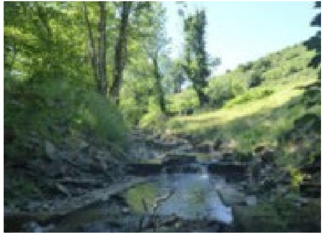
Tarff Creamery Weir after removal
