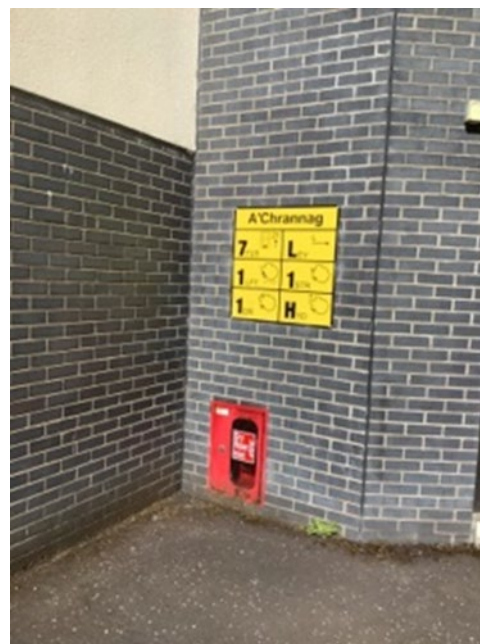
Figure 4: Indicator plate in place on the block shown in figure 2 Source: HMFSI
