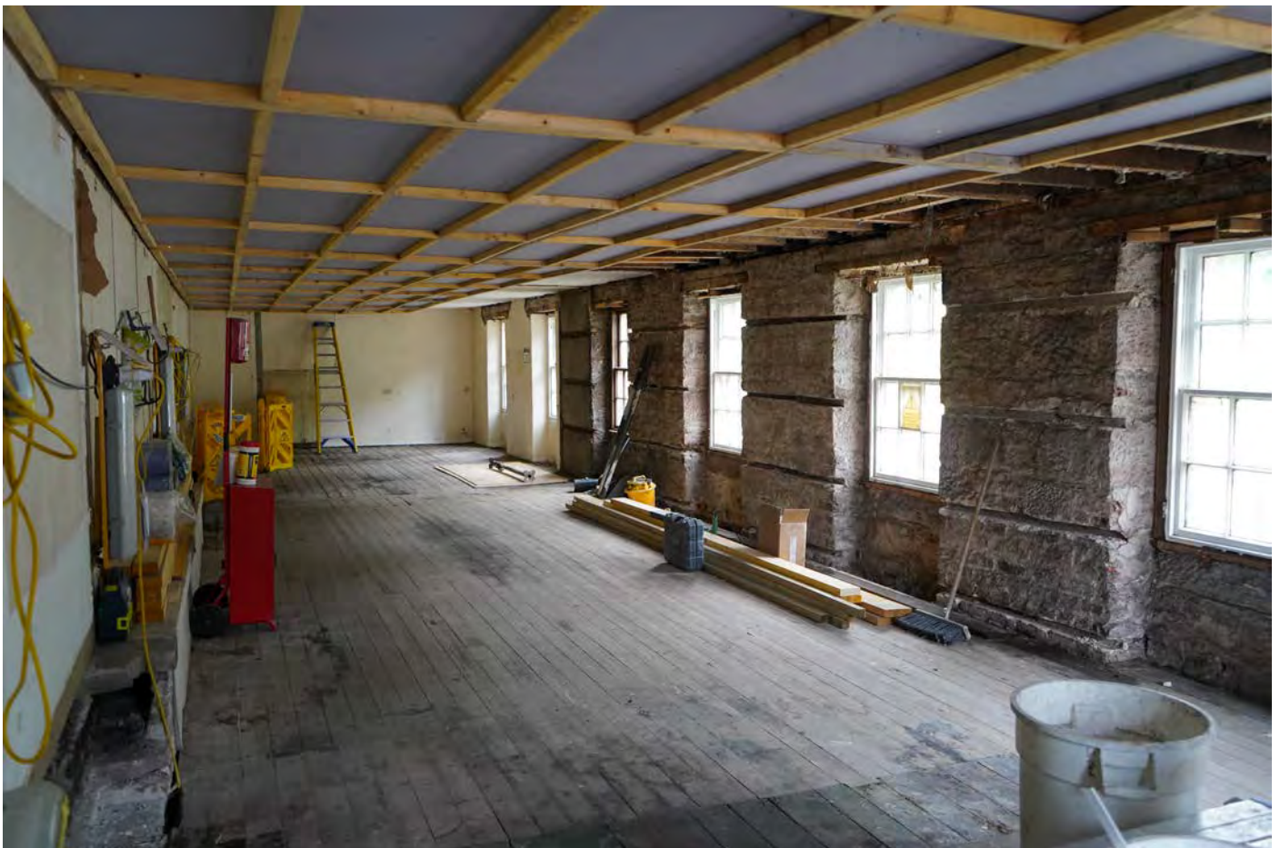
Bothy Building Interior - strip out completed - MAY 2022
