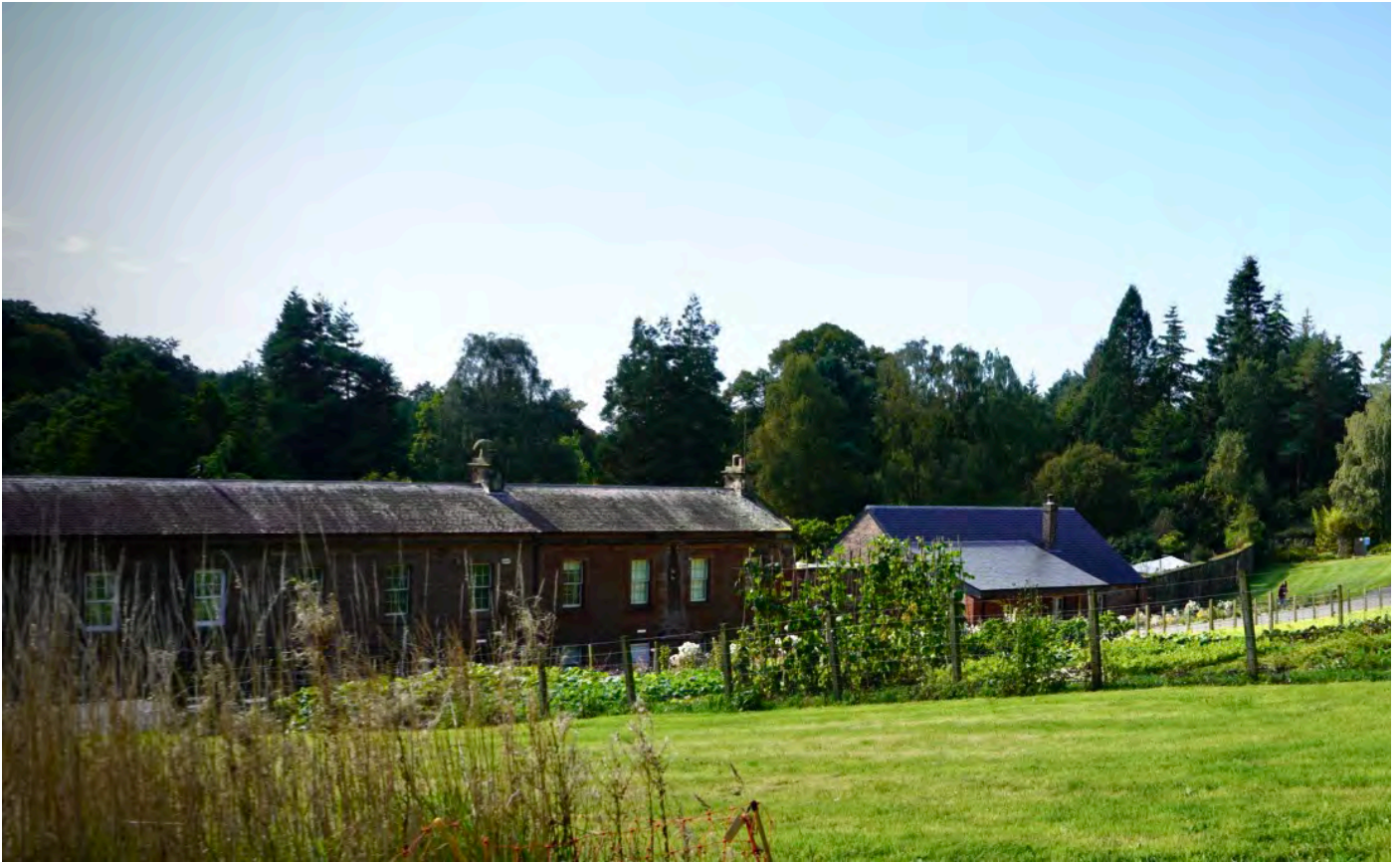
Bothy Building Exterior - SEPTEMBER 2022
