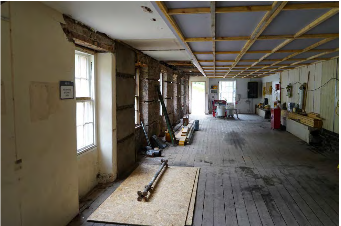
Bothy Building Interior - strip out completed - MAY 2022
