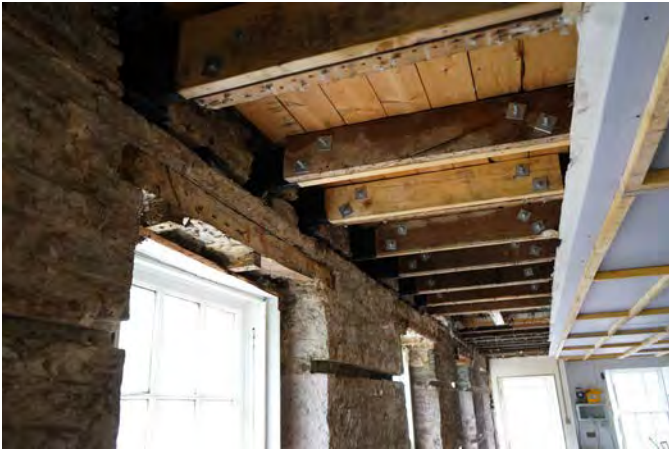
Bothy Building Interior - joist repairs due to dry rot - MAY 2022
