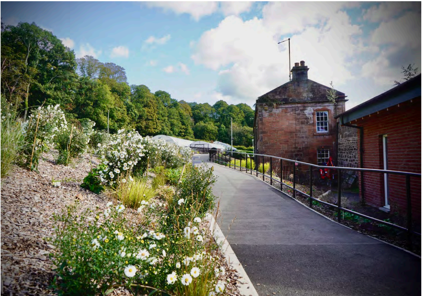
Bothy Building Exterior - SEPTEMBER 2022
