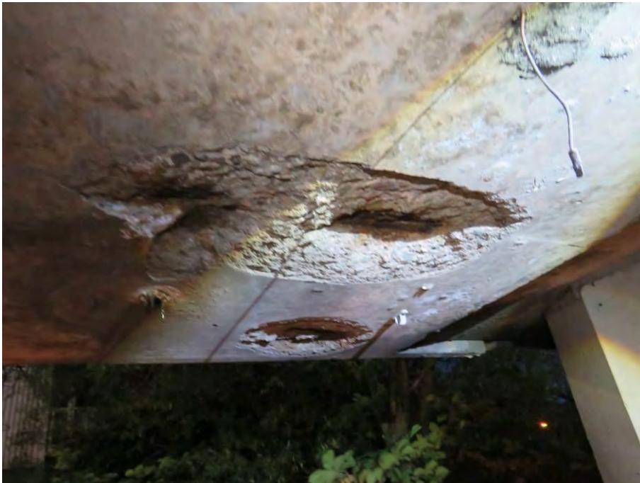
Photo 17 – Localised spall exposing reinforcement at IS6 half joint and span 6 bridge deck
