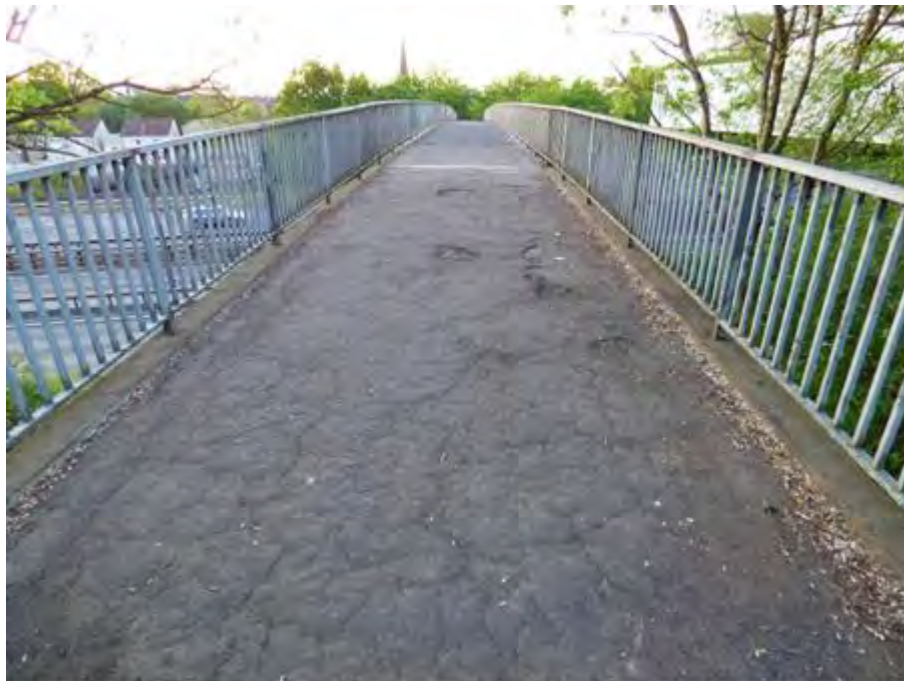
Photo 19 – Deep cracks and potholing to span 5 surfacing
