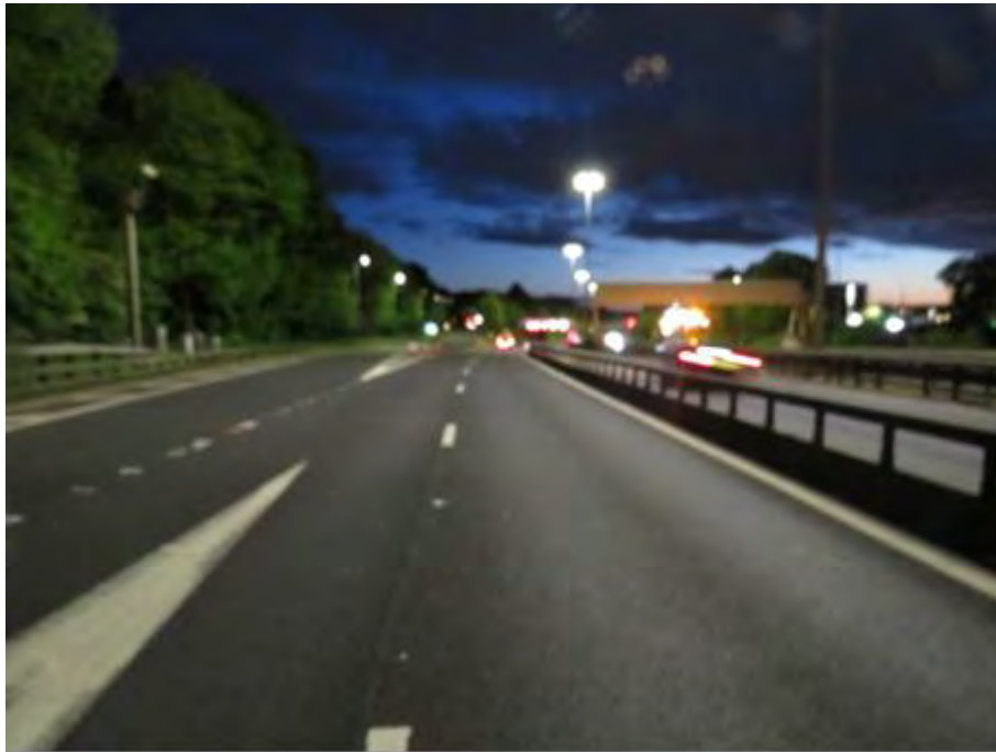
Photo 3 - VIEW LOOKING UPLINK M8
