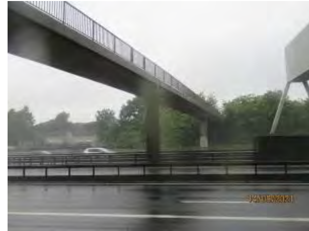
General view of RHS
