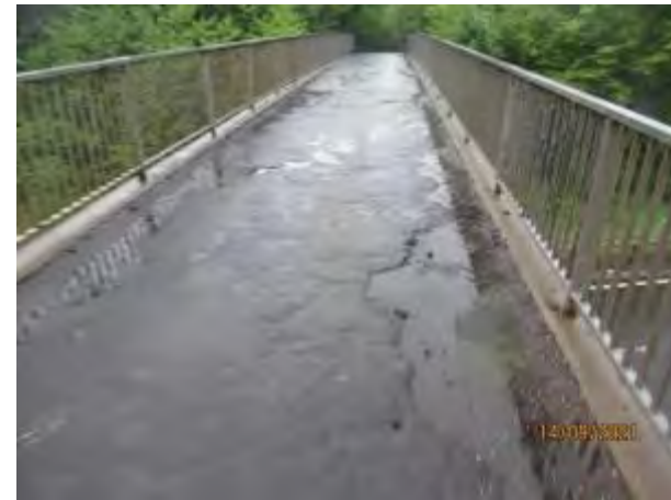
General view of adopted downlink
