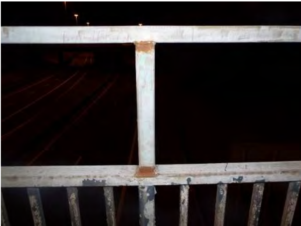
Photograph No.9 - (Typical) Existing paint system is beyond its useful life span. All paint coats failed.
