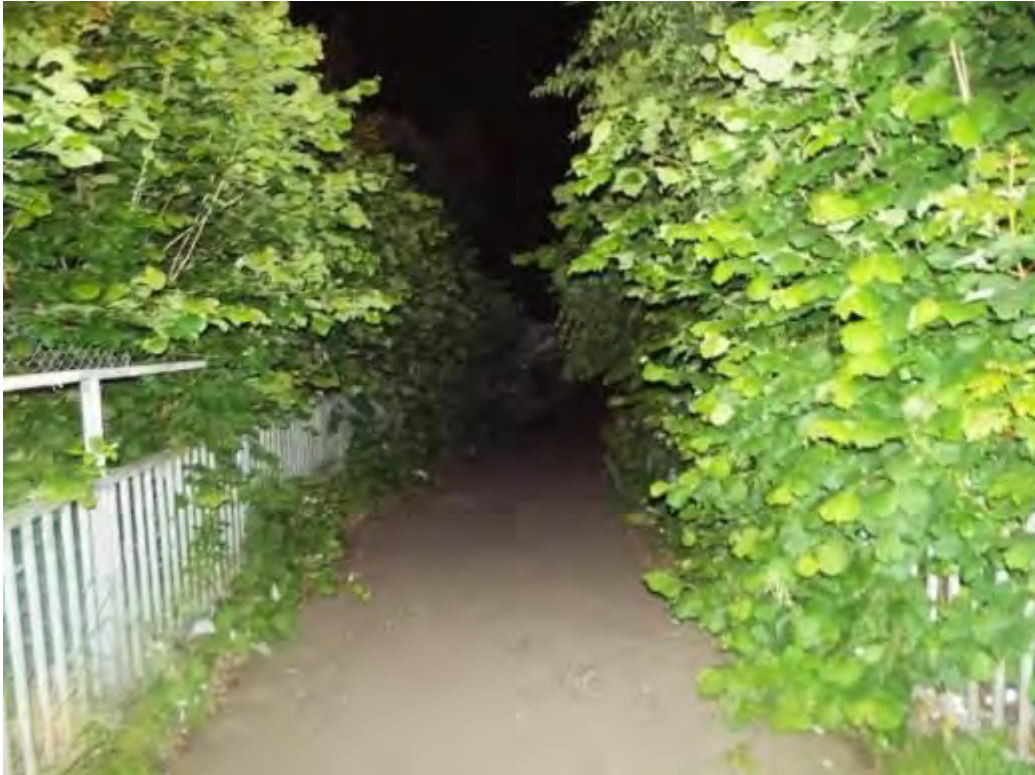
Photograph No.66 - Vegetation growth encroaching on both parapet rails behind ESP 1.
