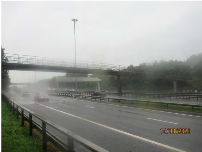
General view of RHS of structure
