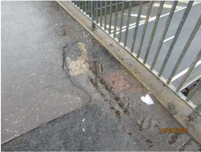
Photo 9 – Gully's completely blocked with debris
