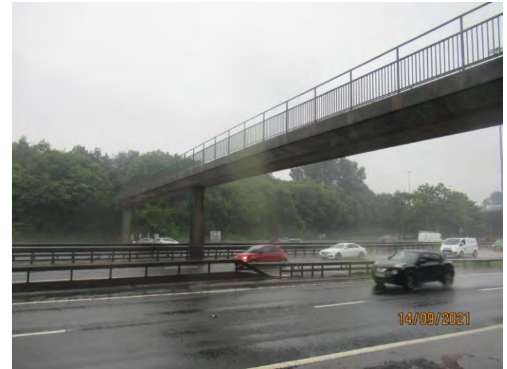
General view of LHS of structure
