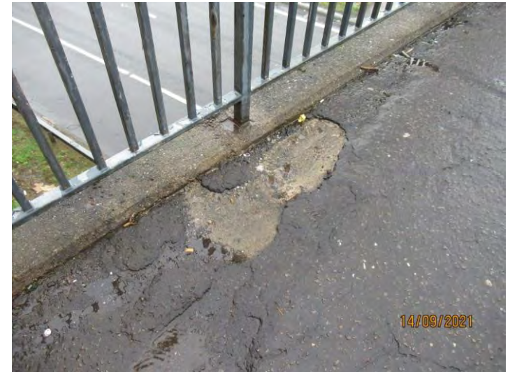
Photo 12 – Break up of footway
