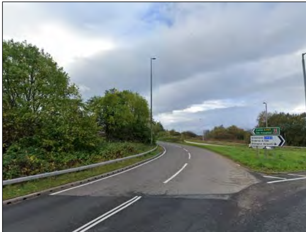
Figure 4-6 – St James Interchange Roundabout Exit to A737 On-Slip
