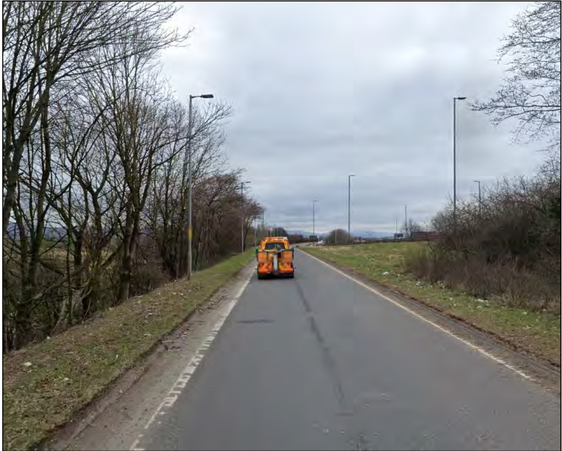
Figure 5-3 – Lincrive Junction Northbound On-Slip
