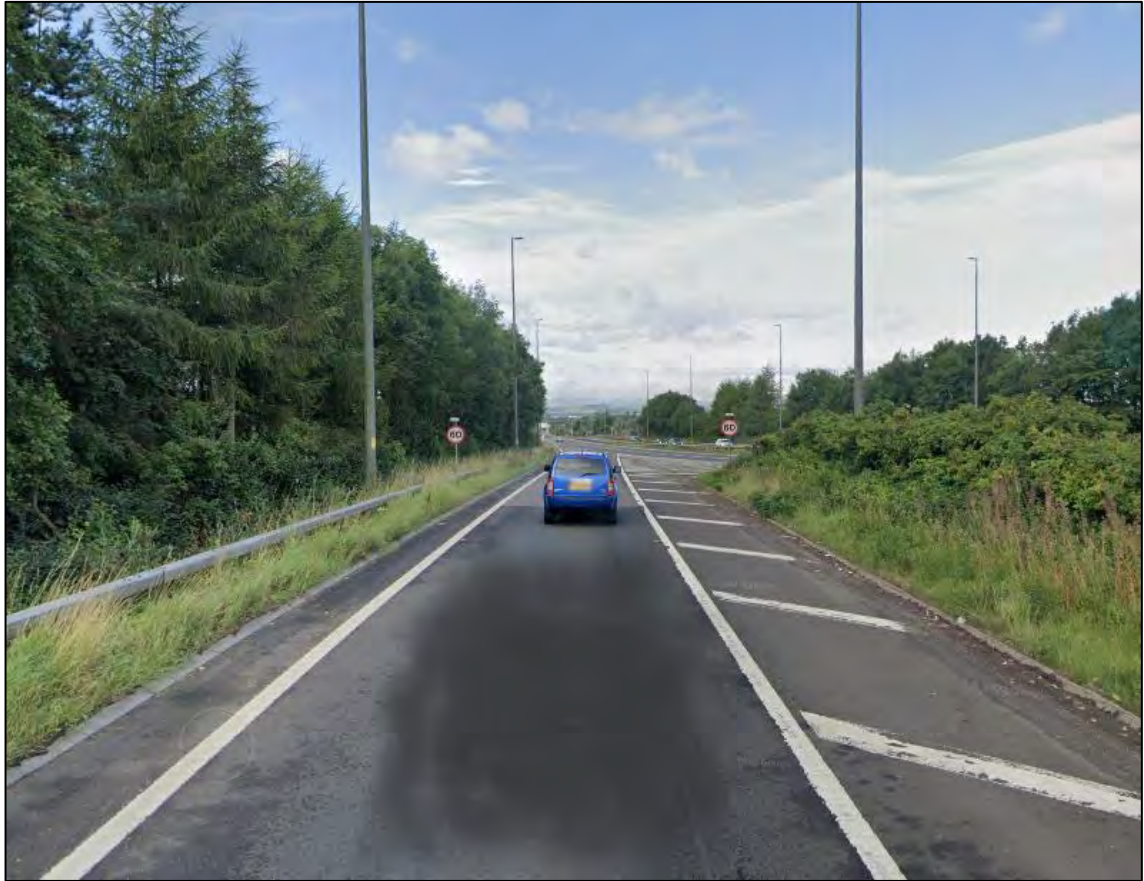
Figure 4-7 – St James Interchange On-Slip Approach to A737 Mainline Merge
