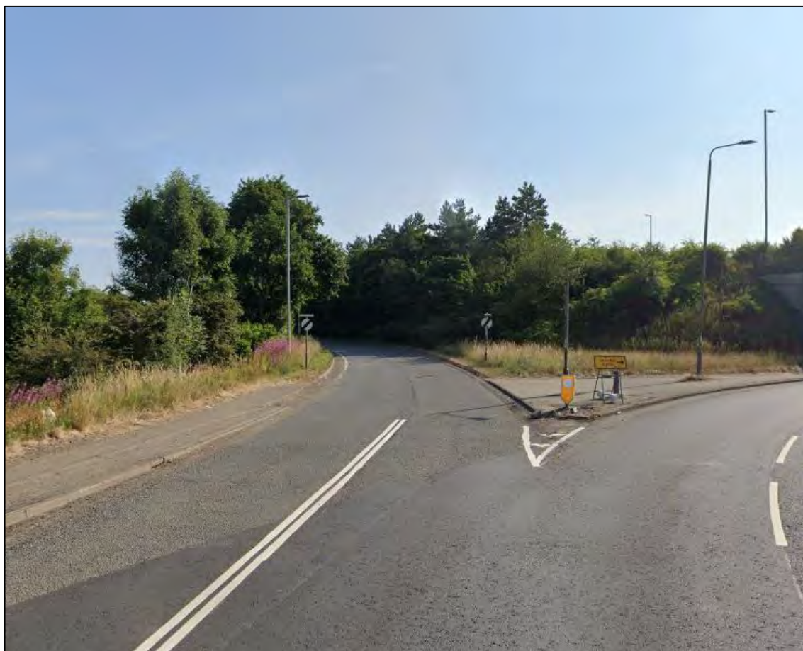
Figure 5-2 – Linclive Junction Northbound On-Slip Entry
