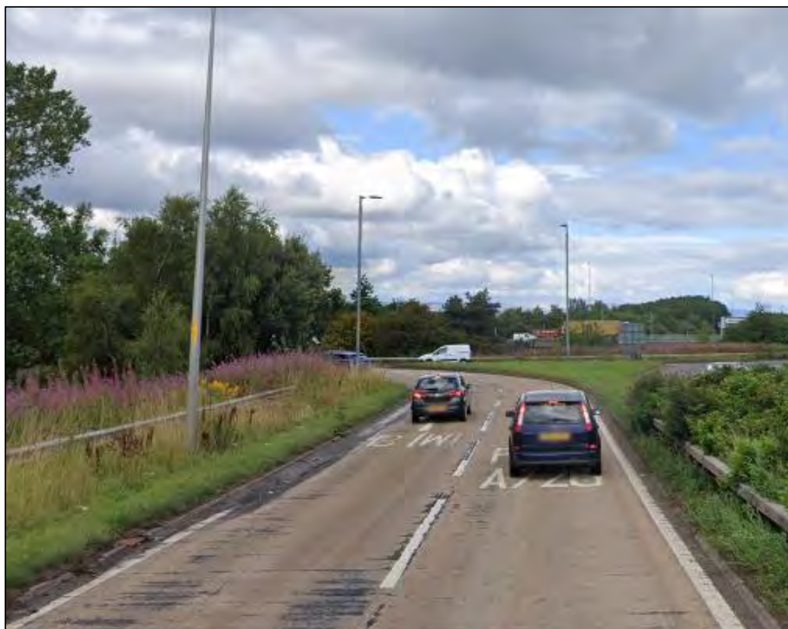
Figure 4-5 – A737 Northbound Off-Slip Approaching St James Interchange Roundabout View
