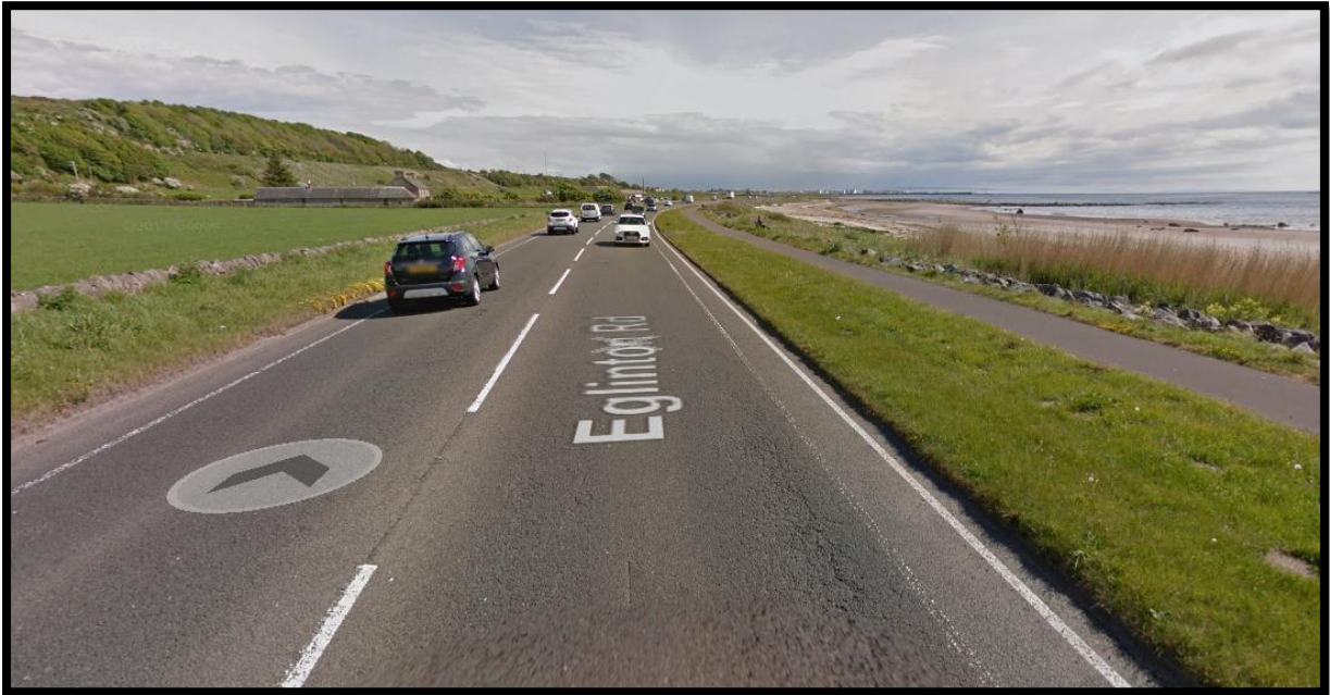
Southbound Approach at 215m
