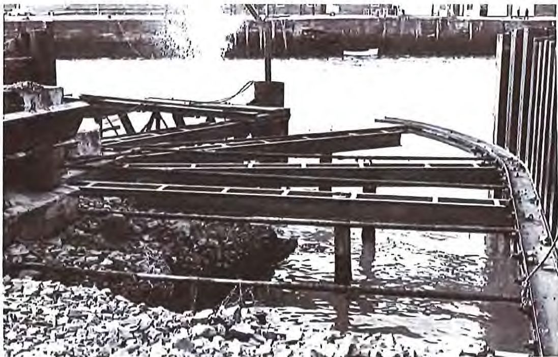
Figure 4 Photograph during construction (dated 1975)
