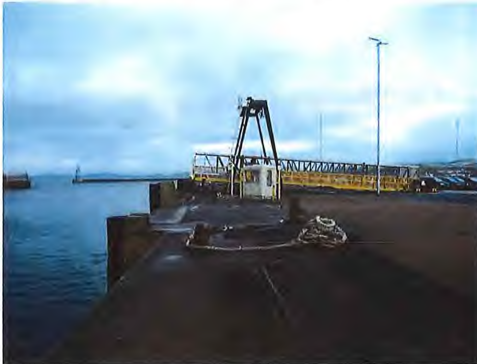
Photo 12 – General view along the ferry berth at Ardrossan
