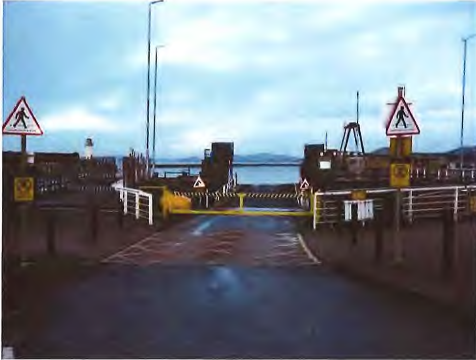
Photo 6 – The linkspan approach at Ardrossan
