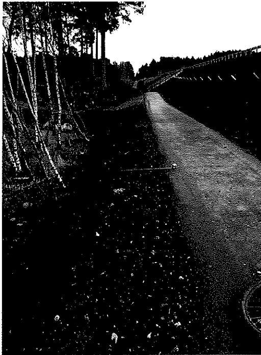
Problem 3.27 – NMU Track at Ch. 3850
