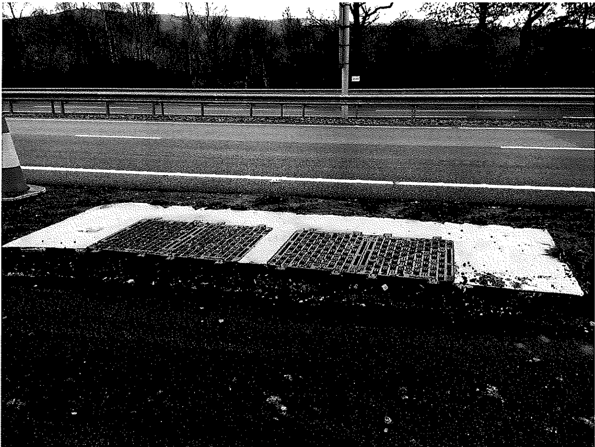
Problem 3.7 – Example of Rasied Service Covers
