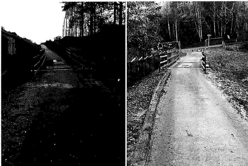
Problem 3.3 – Fencing at ST01
