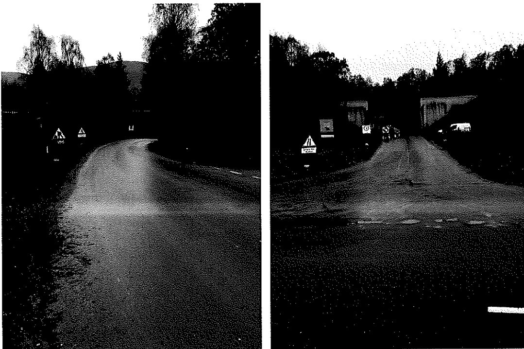
Problem 3.1 –No Signage Provided to Identify NMU Route
