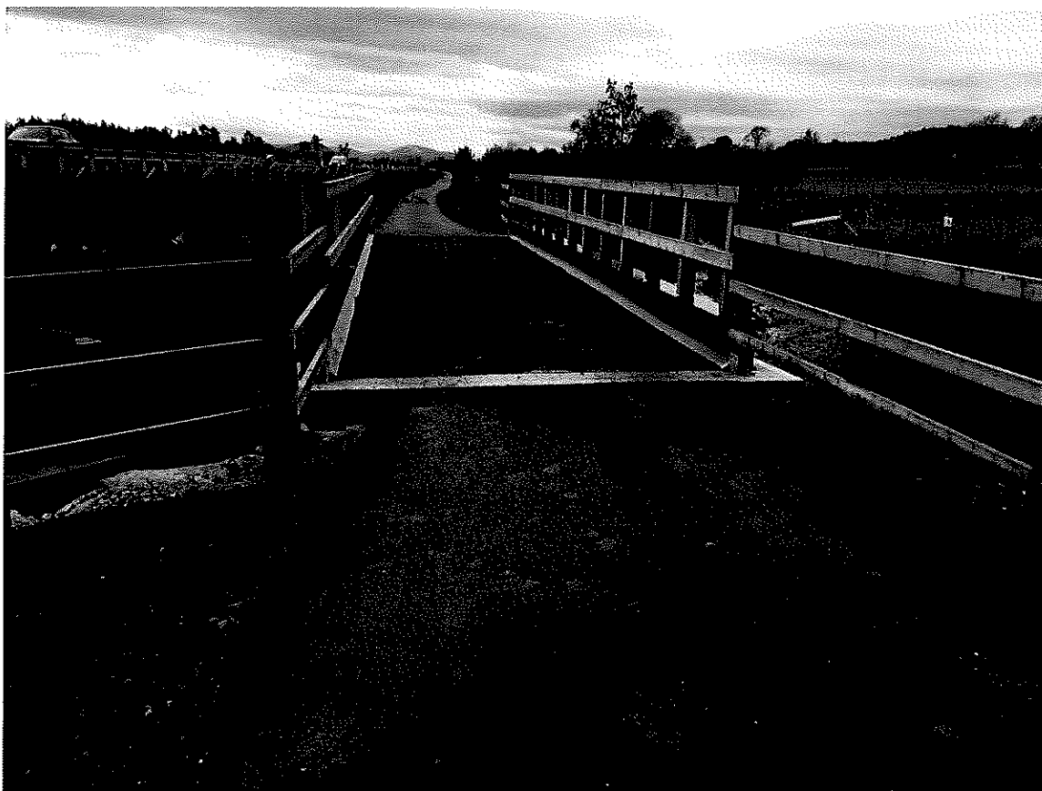
Problem 3.16 – NMU Watercourse Bridge Ch.3125 Approx.
