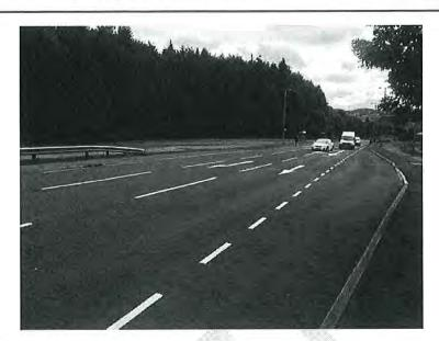
Summary: There is clear evidence of vehicles overrunning the existing central hatching when turning right into the B6359 road. The scheme will introduce a refuge island where the markings currently exist resulting in the potential of it being stuck by vehicles.
