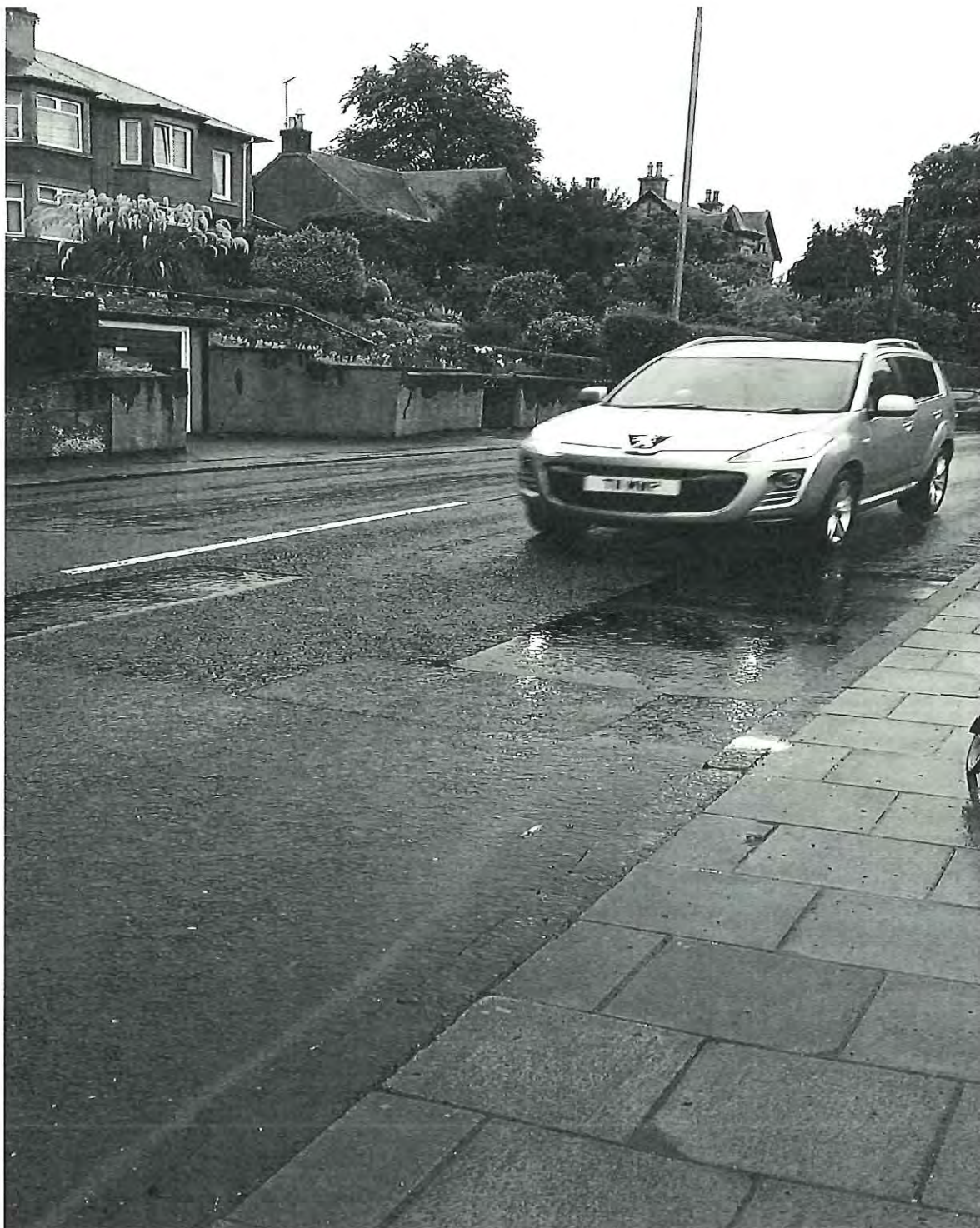
11039/36 ch298m end of scheme old patches and fretting
