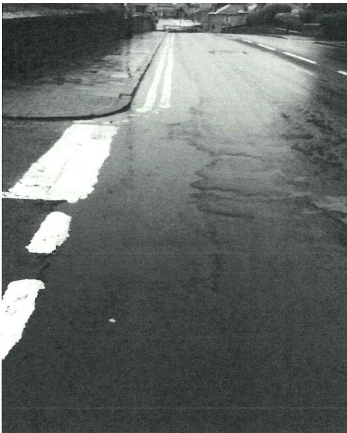
11039/36 ch95m SB starting to rut and fretting
