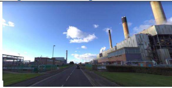
Image 4 - A904 looking North West
