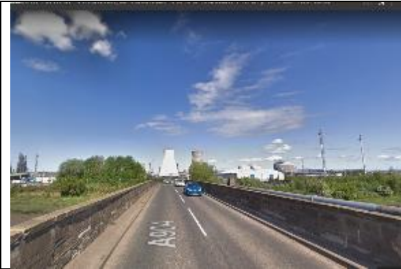
Image 1 - At Avon Bridge on A904
