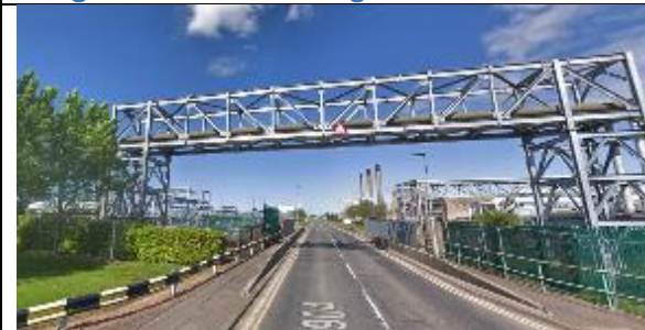
Image 3 - Existing pipe bridge
