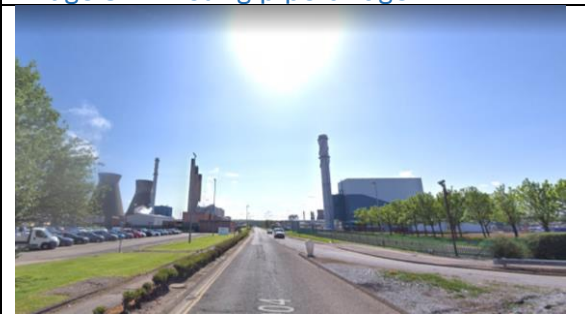
Image 5 - A904 Inchyra Roundabout looking South East
