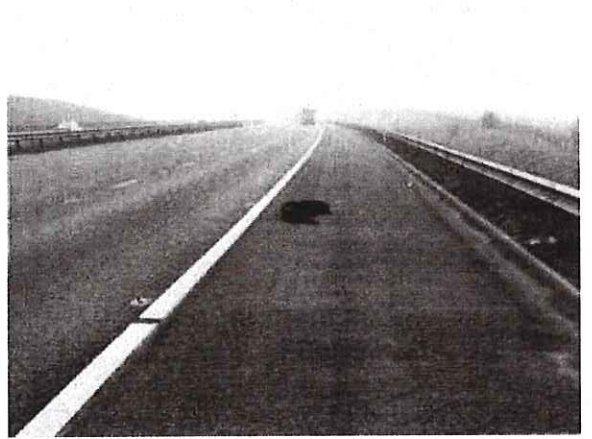
DBHS Debris in hard shoulder
