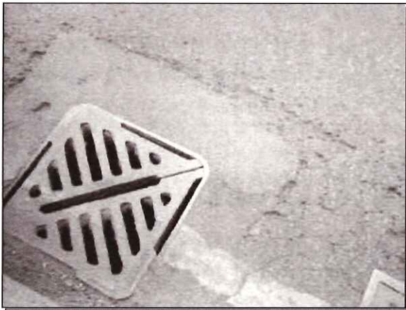
PACK Patch adjacent cracking
