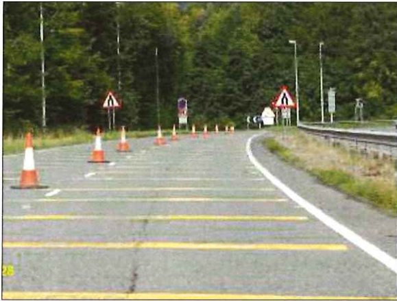
SRJT Surfacing Joints
