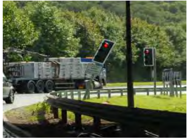
PLCD Condition poles/caps/heads/boards
