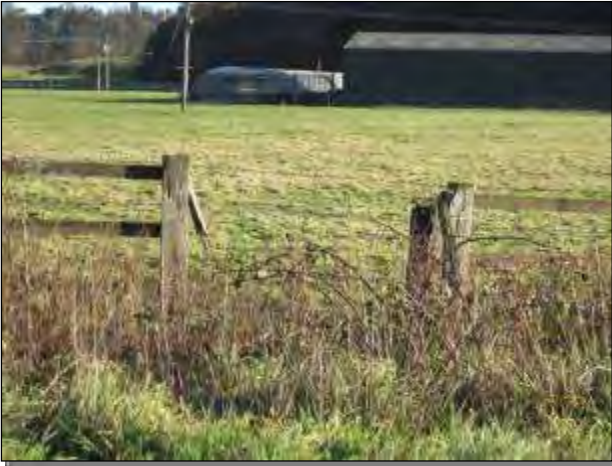
RWDF Rotten wood fence
