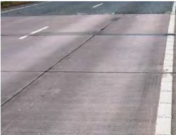
03 Surface: Concrete (code 3)
