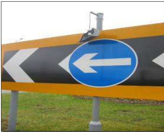
COEL Electrical condition
