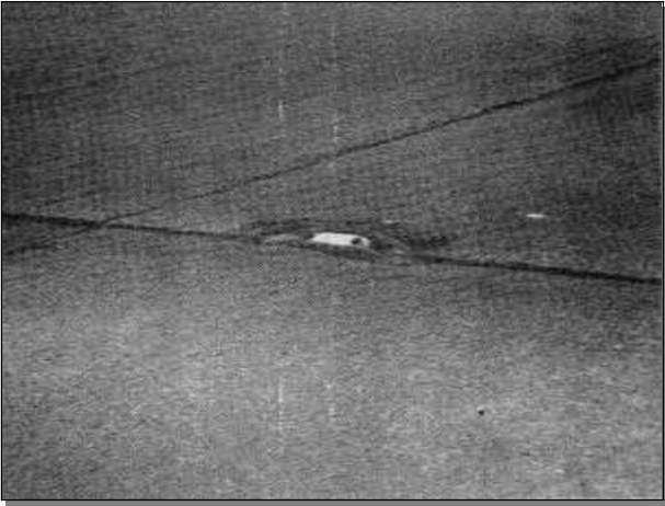
LCAS Loose Catseye casing
