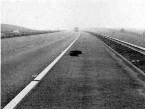
DBHS Debris in hard shoulder
