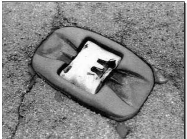
MISR Missing Reflector
