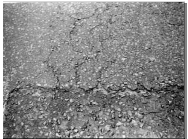
TACK Trench RI – adjacent cracking
