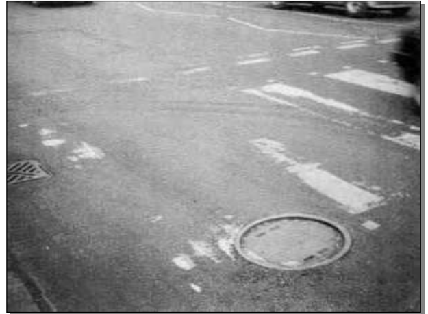
ICLV Difference in component levels
