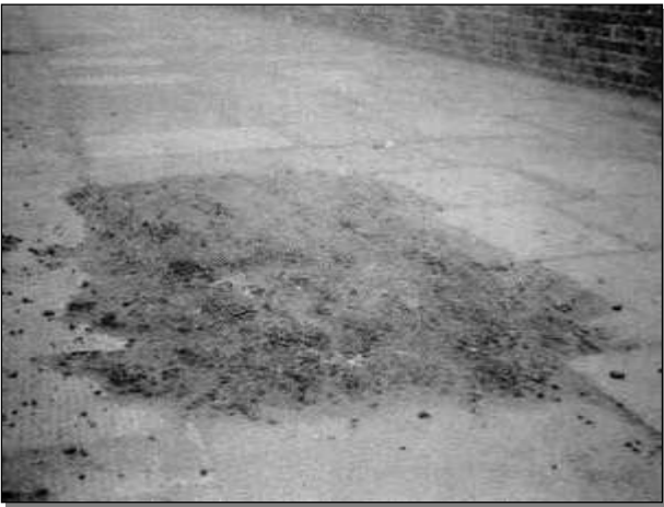
FDLV Failed Patch – difference in level
