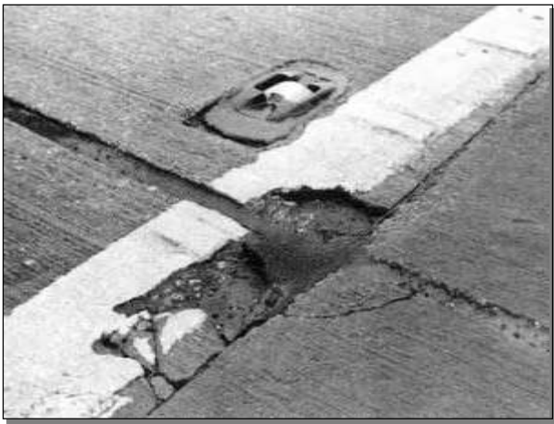
DSPL Deep spalling at joints
