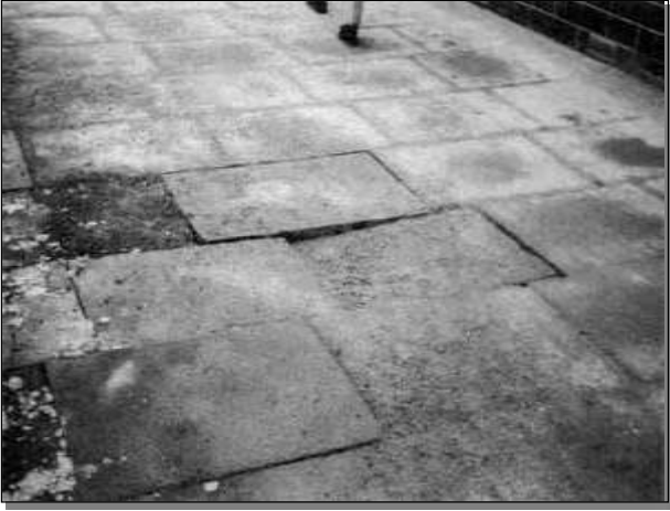
SLPF Slab profile – uneven/trips
