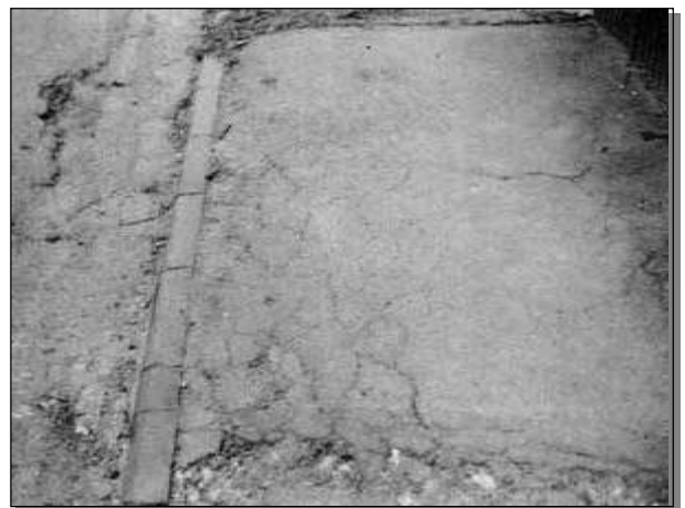
BECK Bituminous Surfacing – Extensive Cracking
