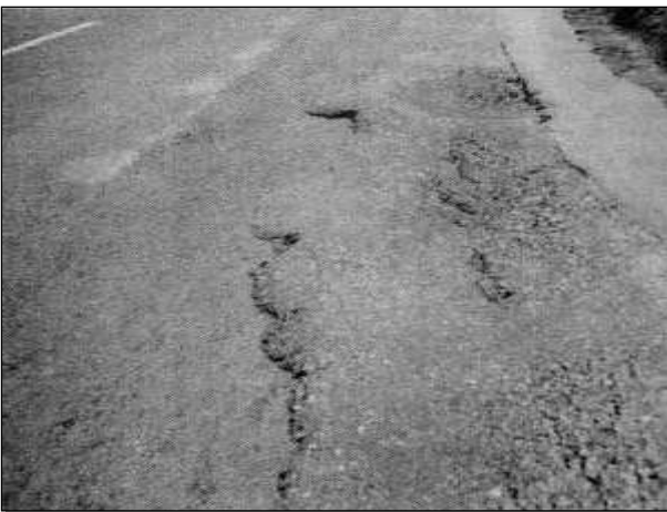
PDLV Patch – difference in level
