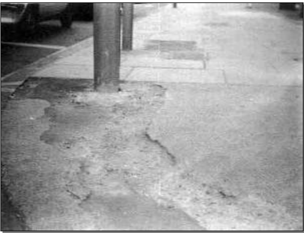
RLMT Trench RI – loss of material
