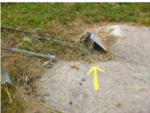
LOSA Loose Anchor
