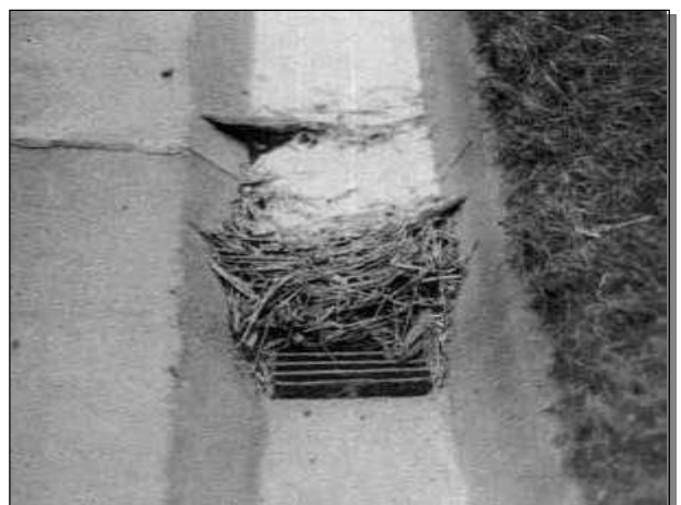
IMWF Impeded water flow
