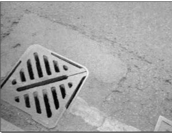
PACK Patch adjacent cracking
