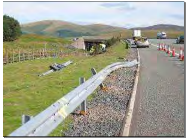
DAMM Damaged Deformed Fence/ Barrier
