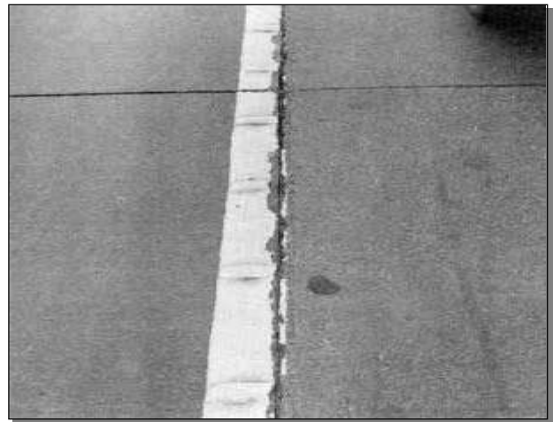
OLJT Opening of longitudinal joint
