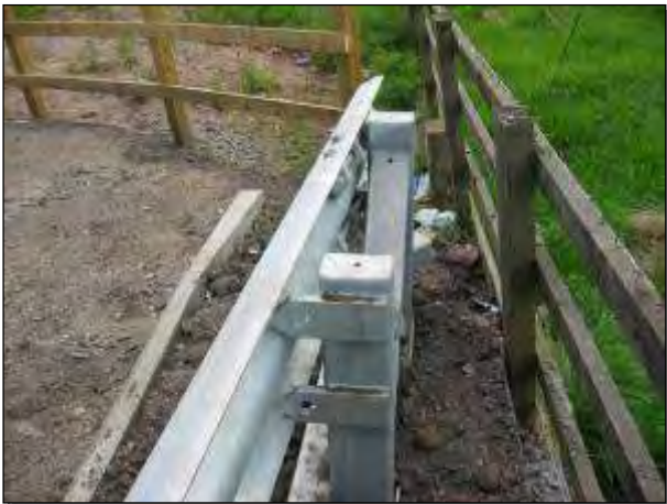
NTEN Incorrect or no tension (metal fence)
