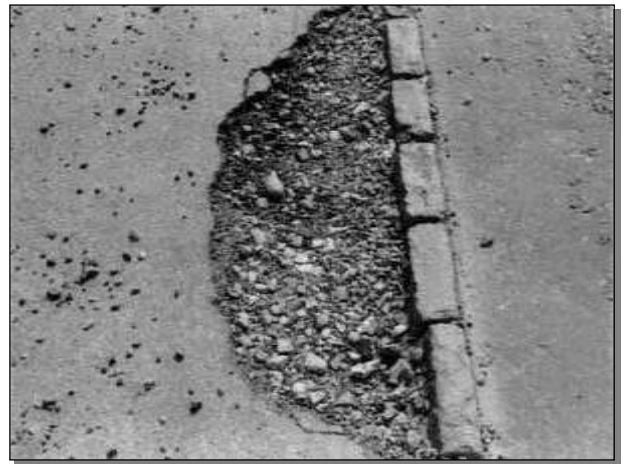
BPOT Bituminous surfacing – potholes
