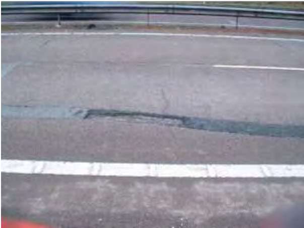
OVSD Failed overbanding / sealed cracks
