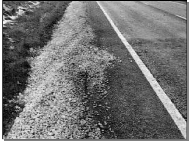
FMDS Filter Material displaced
