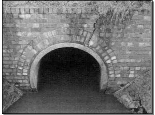
CRCK Cracking
