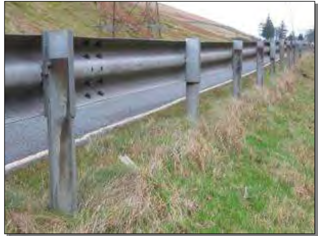
CMTP Corroded – metal post (fence / barrier)
