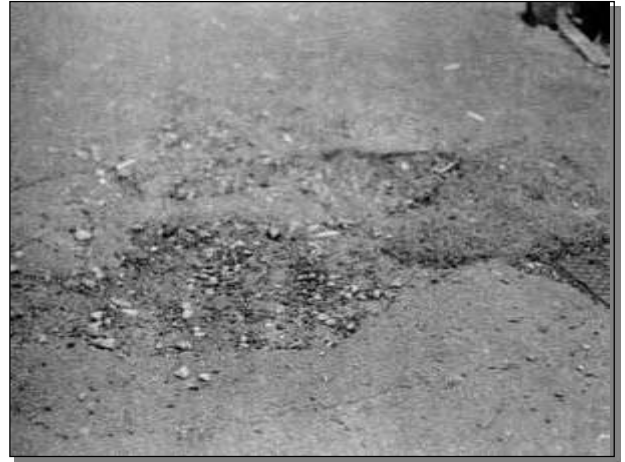
FLMT Failed Patch – loss of material
