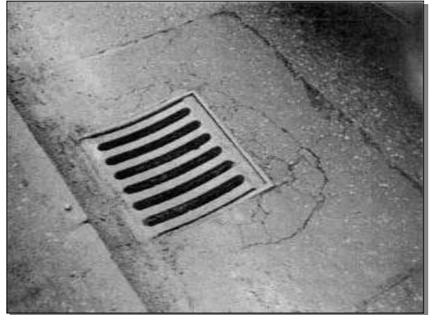
CKIR Cracking around ironwork
