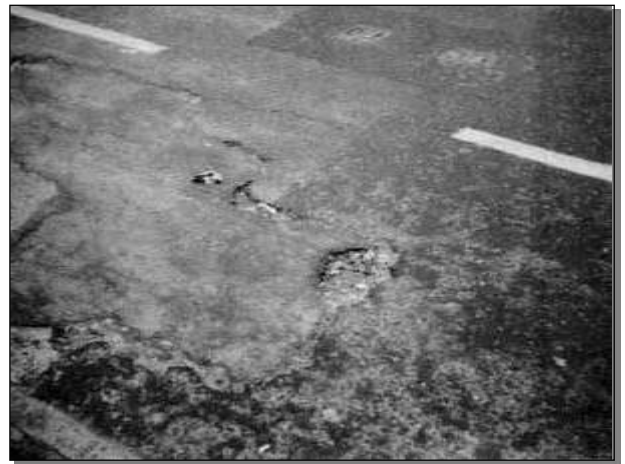
PLMT Patch – loss of material
