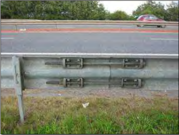
LTEN Loose tension bolt
