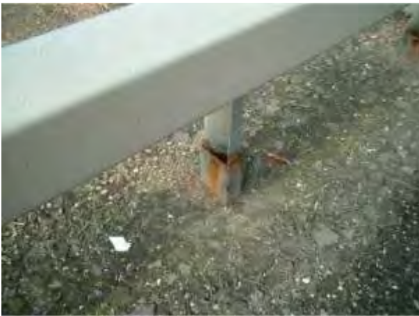
CMTP Corroded – metal post (fence / barrier)
