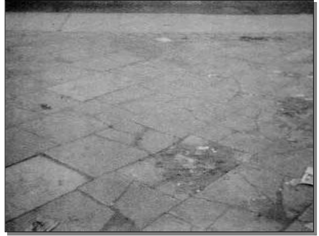
SLCK Slab Cracking
