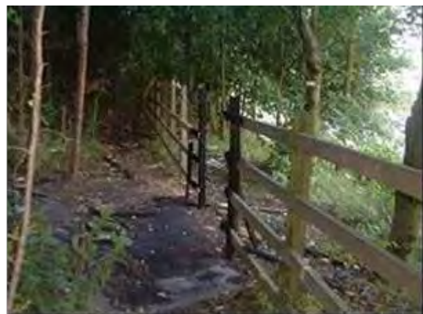
RWDP Rotten - Wood Post (Fence/ Barrier)
