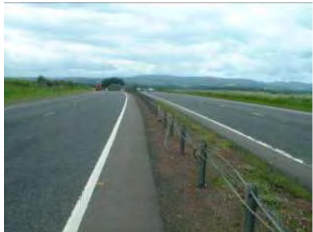
CORT Incorrect Tension
