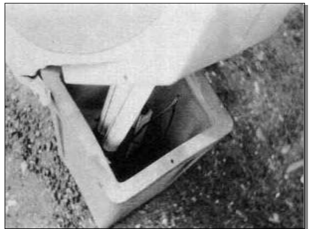
EXPW Exposed wiring
