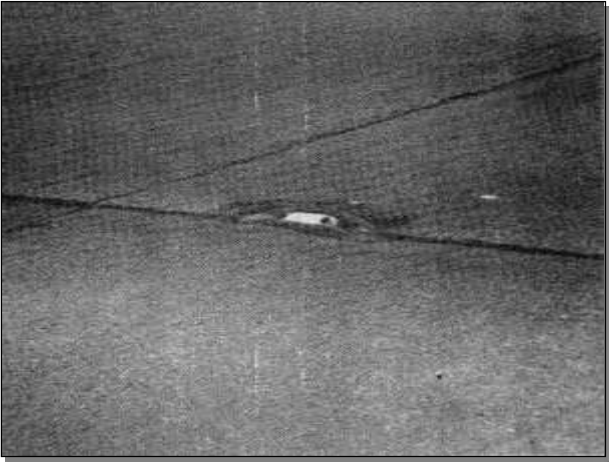
LCAS Loose Catseye casing
