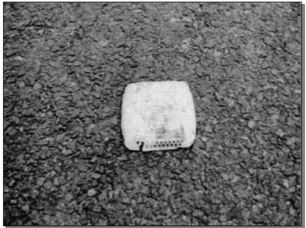
DAMS Damaged stud
