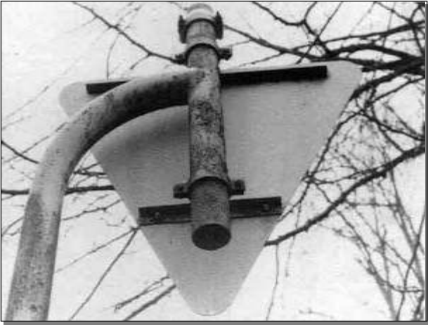
SFCO Surface corrosion
