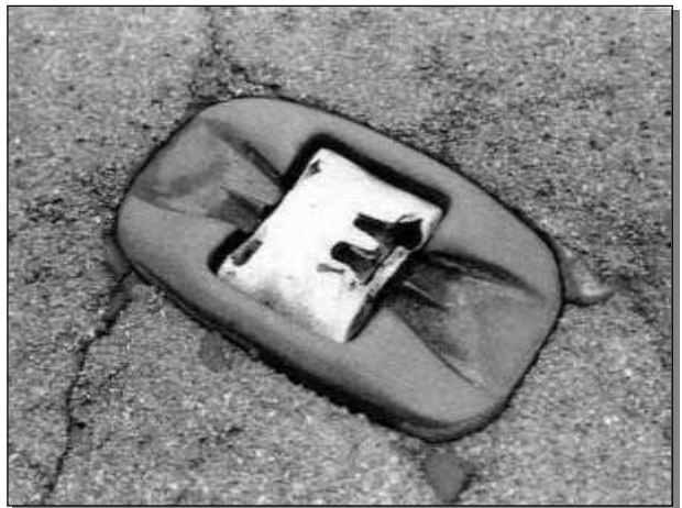
MISR Missing Reflector
