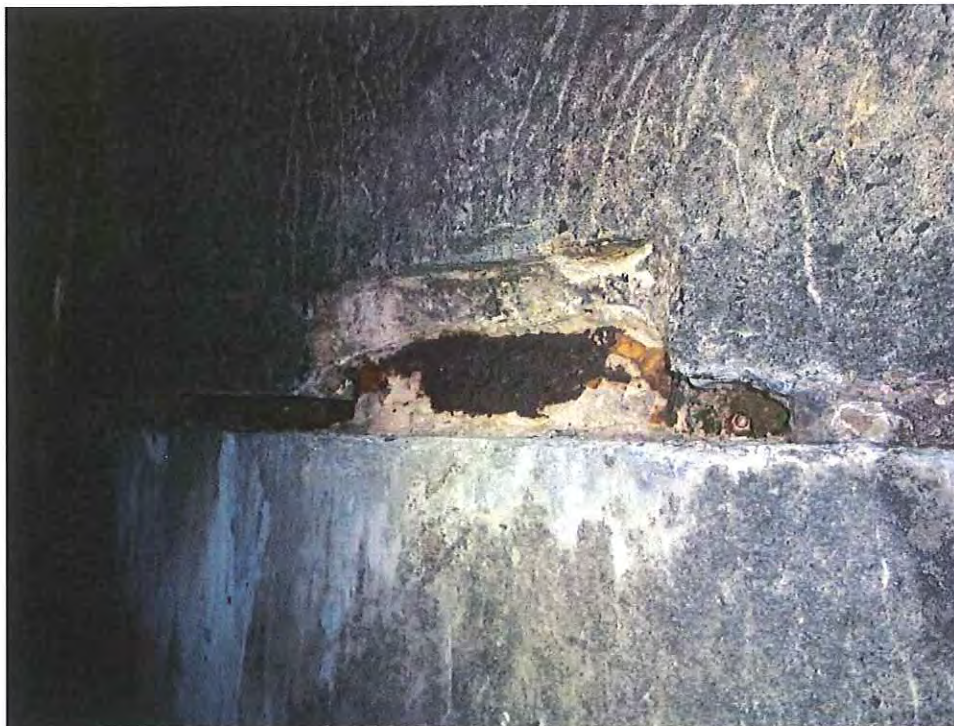
Photo D13 – DEFECT: - Wingwall lifting point exposed
