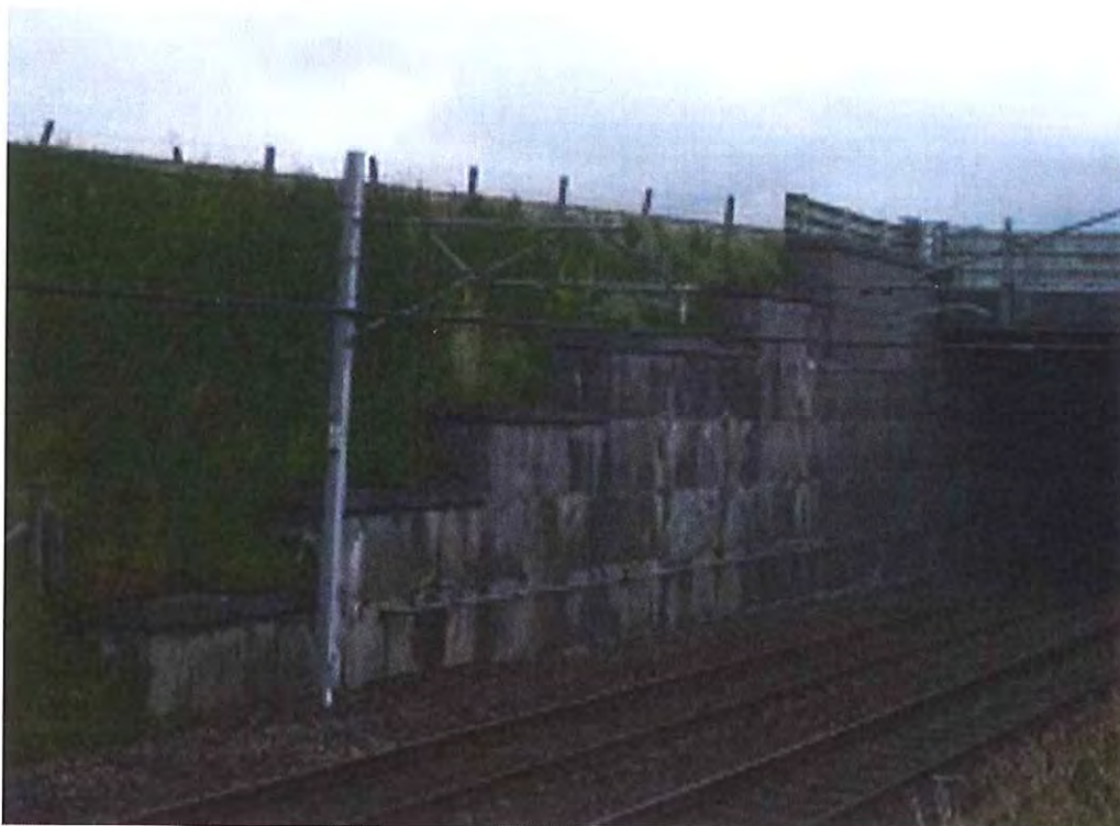
Photo G10 -RHS Downlink WINGWALLS
