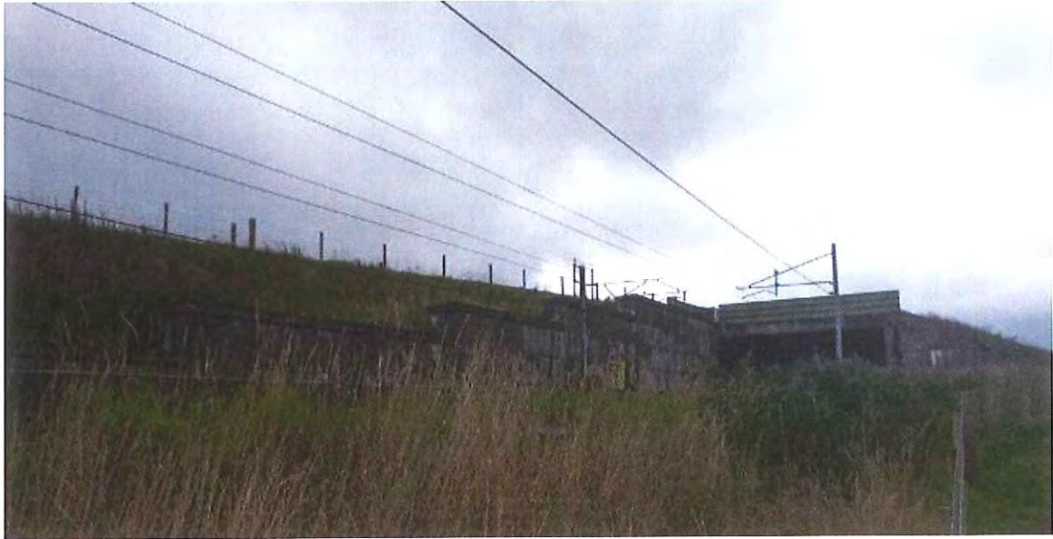
Photo G7 –LHS Uplink WINGWALLS
