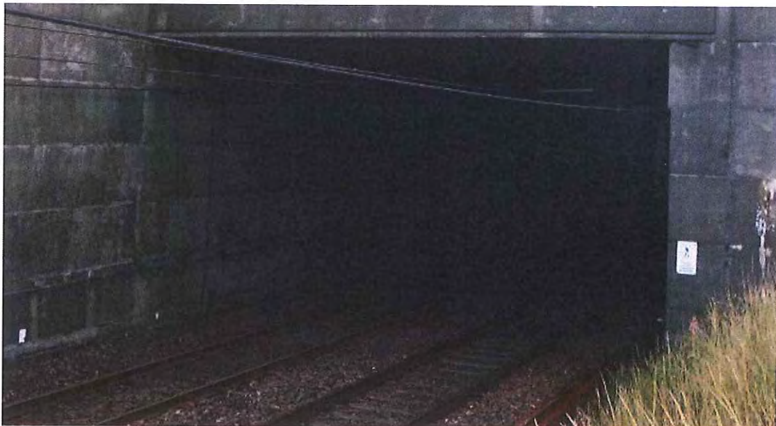
Photo G6 - Downlink ABUTMENT
