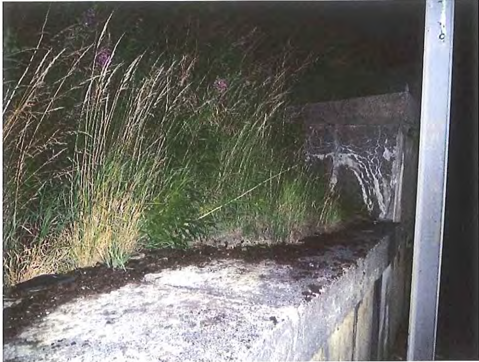
Photo D17 – DEFECT: - Wingwall – Polysulphide joint material breaking out along wing wall/abutment joint
