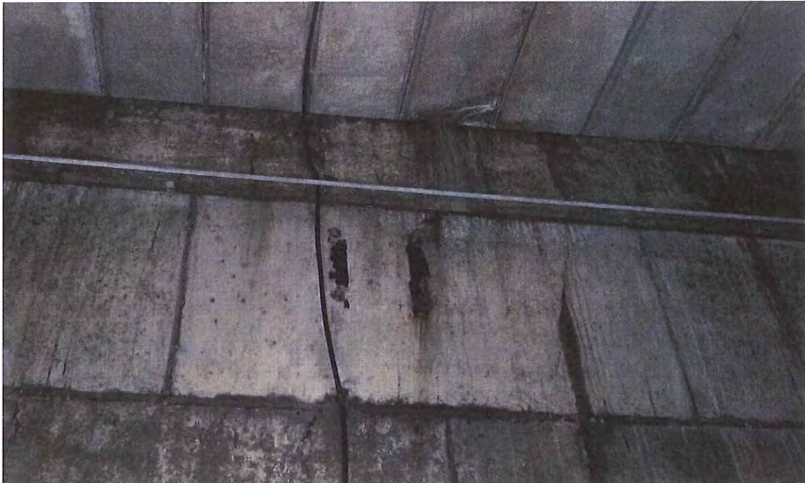
Photo D9 – DEFECT: - Bolts from decommissioned connection remain in abutment
