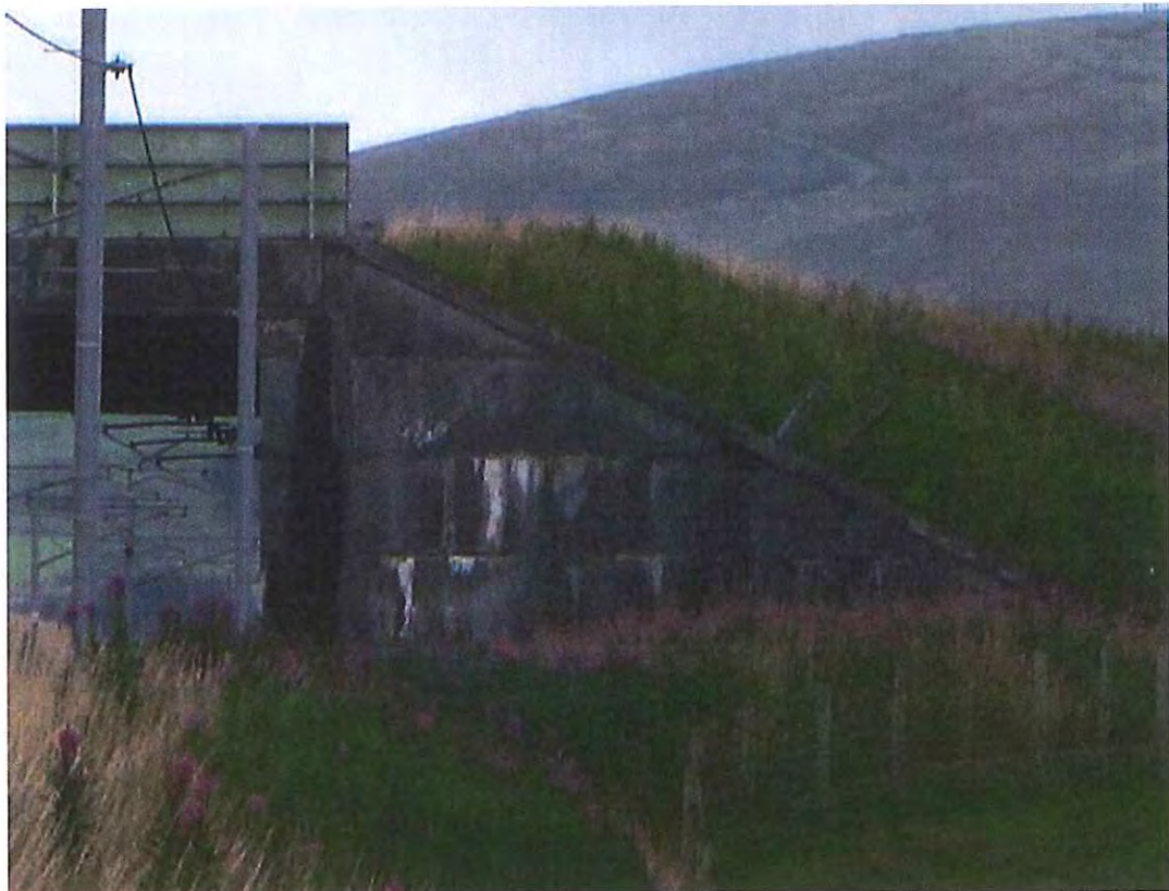
Photo G8 –LHS Downlink WINGWALLS
