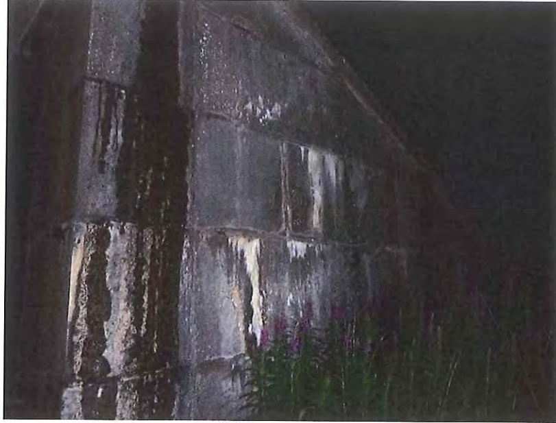
Photo D19 – DEFECT: - Wingwall – Isolated areas of Masonry breaking out, leaking
