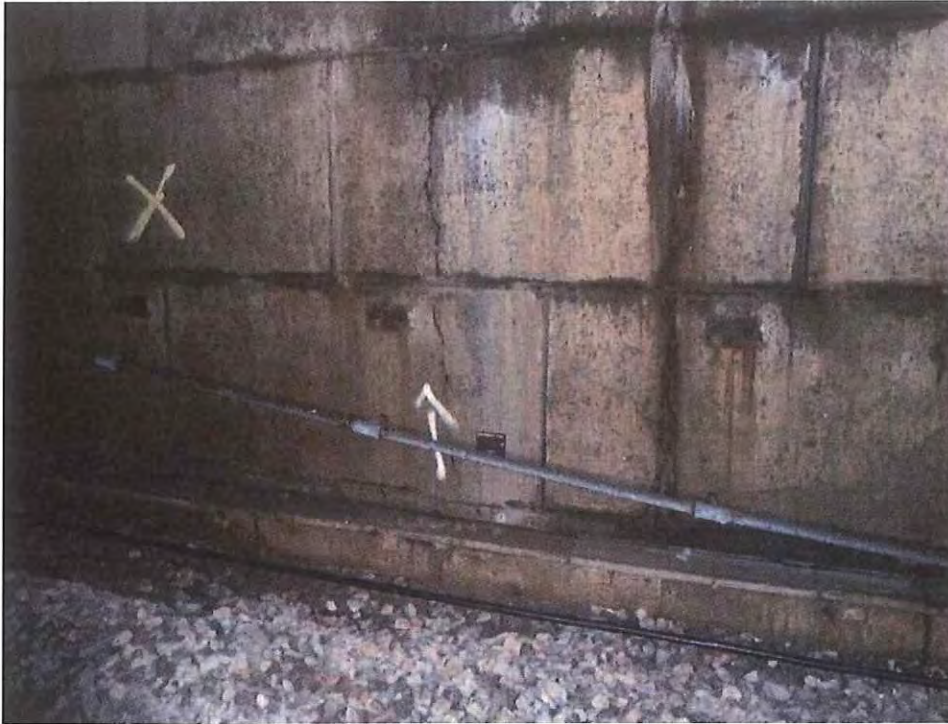
Photo D9 – DEFECT: - Bolts from decommissioned connection remain in abutment
