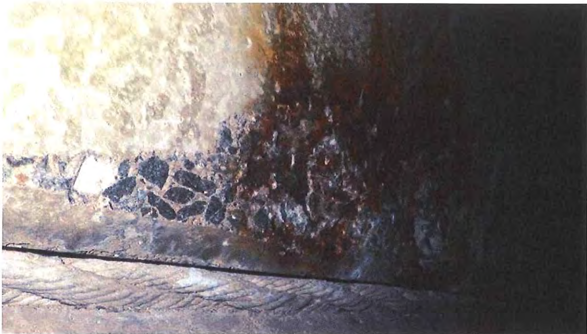
Photo D3 – DEFECT: - Localised spalling of soffit beam concrete – Mid structure near Support 1
