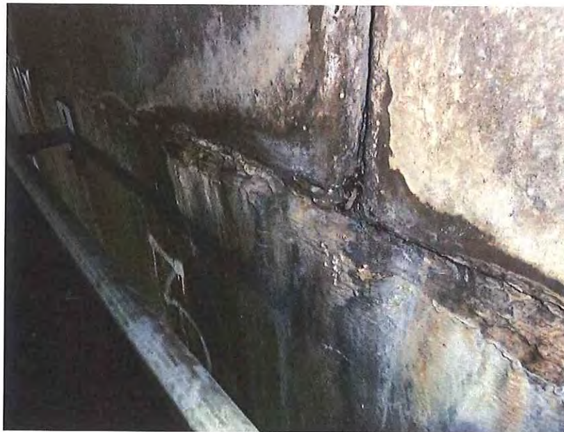
Photo D19 – DEFECT: - Wingwall – Isolated areas of Masonry breaking out, leaking
