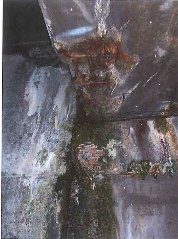
Photo D3 – DEFECT: - Localised spalling of soffit beam concrete – Mid structure near Support 1
