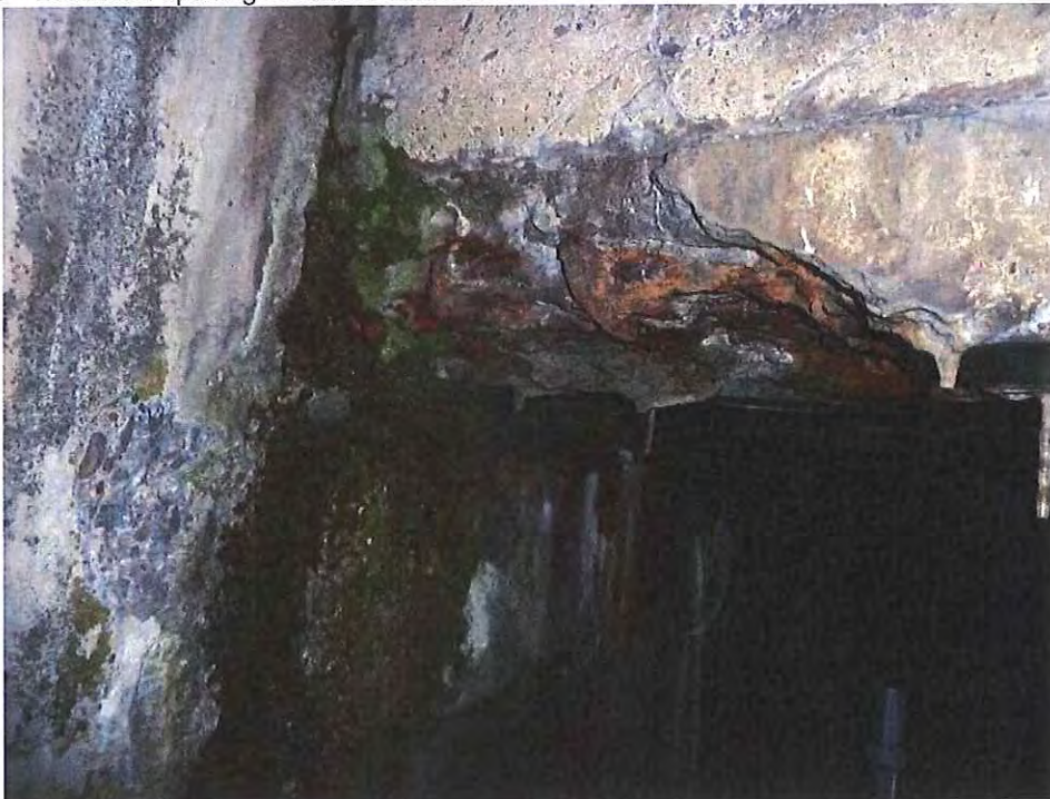
Photo D1 - DEFECT - Localised spalling of soffit beam concrete
