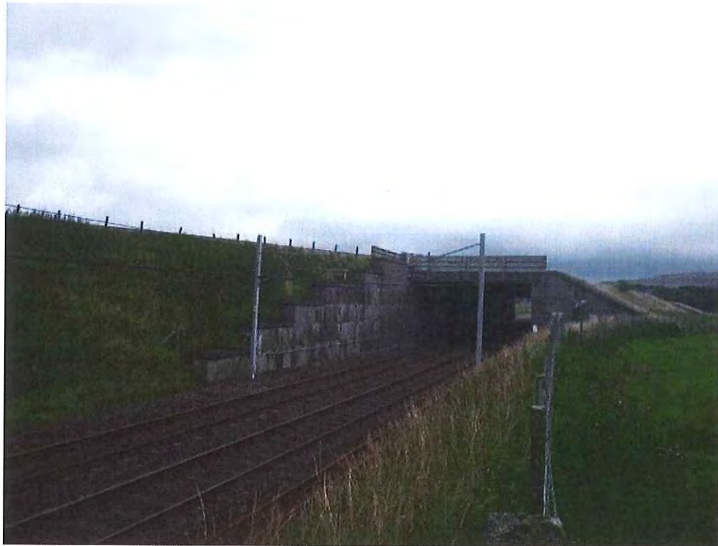
Photo G2 - RHS ELEVATION
