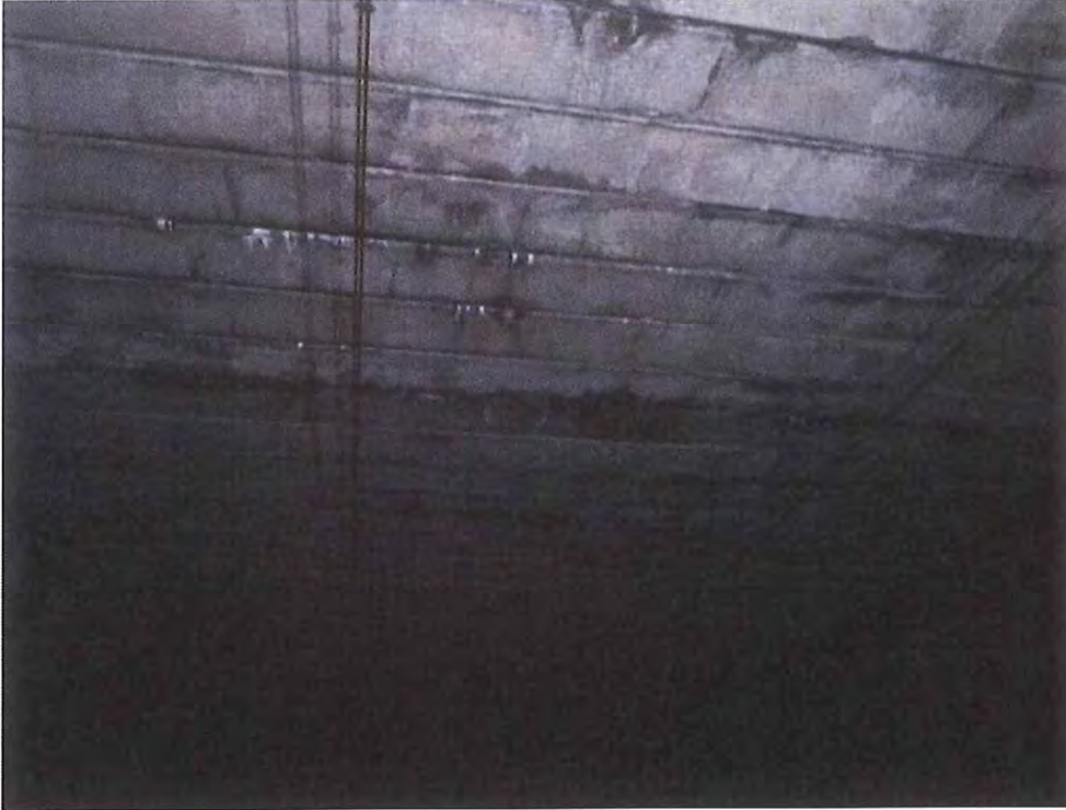
Photo D1 - DEFECT - Localised spalling of soffit beam concrete
