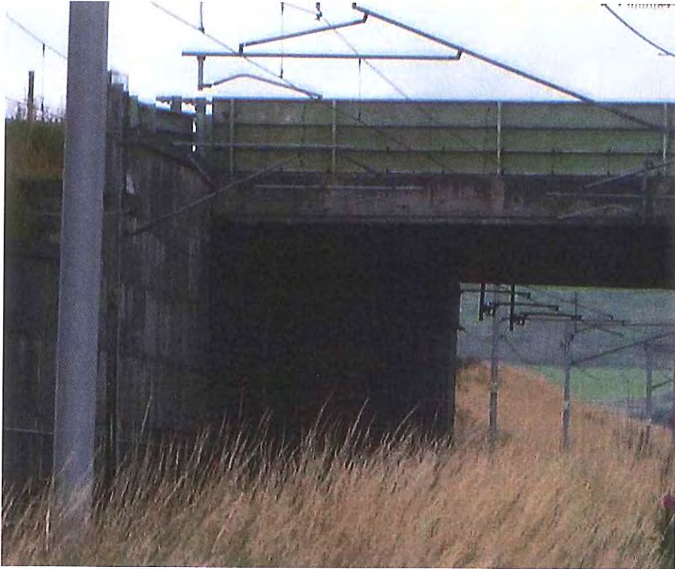
Photo G5 - Uplink ABUTMENT
