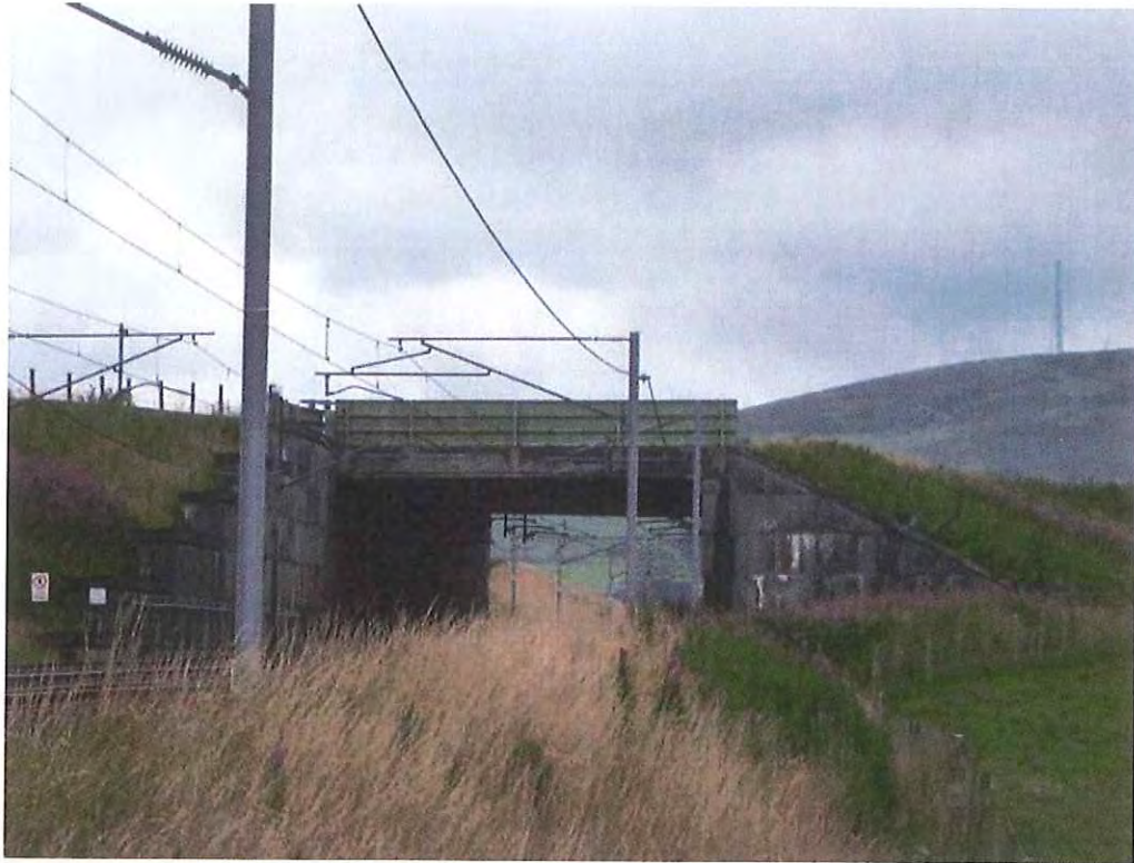
Photo G1 – LHS ELEVATION
