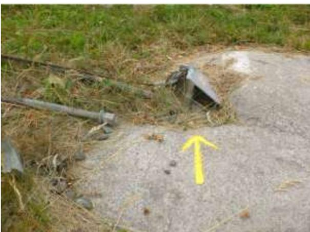
**LOSA** Loose Anchor
