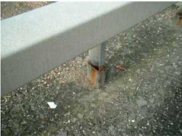
**CMTP** Corroded – metal post (fence / barrier)
