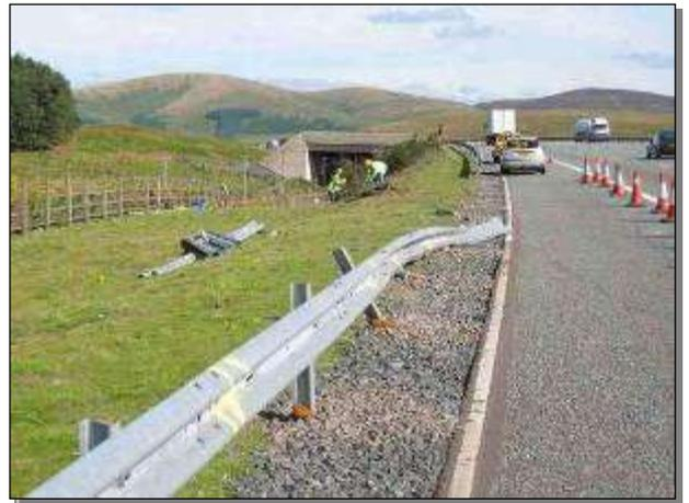
**DAMM** Damaged Deformed Fence/ Barrier
