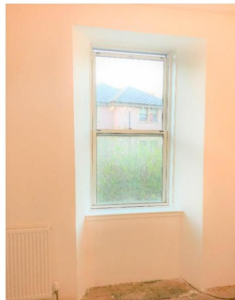
When the installation started, the contractor worked around the property, taking each room one at a time. The work involved temporarily removing radiators, light and plug sockets and attaching 60mm insulation panels. The insulation boards were taped between the joins, skimmed with plaster and painted.
