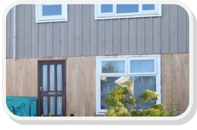
Fig 6. Ply boarding applied to the ground floor, ready for fixing the insulation boards.
