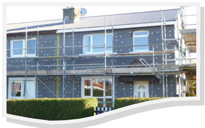
Fig 6. Ply boarding applied to the ground floor, ready for fixing the insulation boards.
