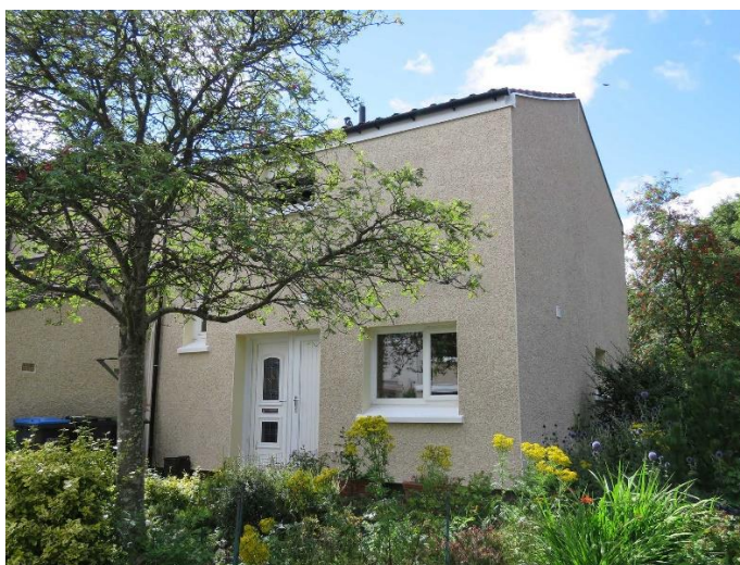
Gillian's home after the insulation was installed
