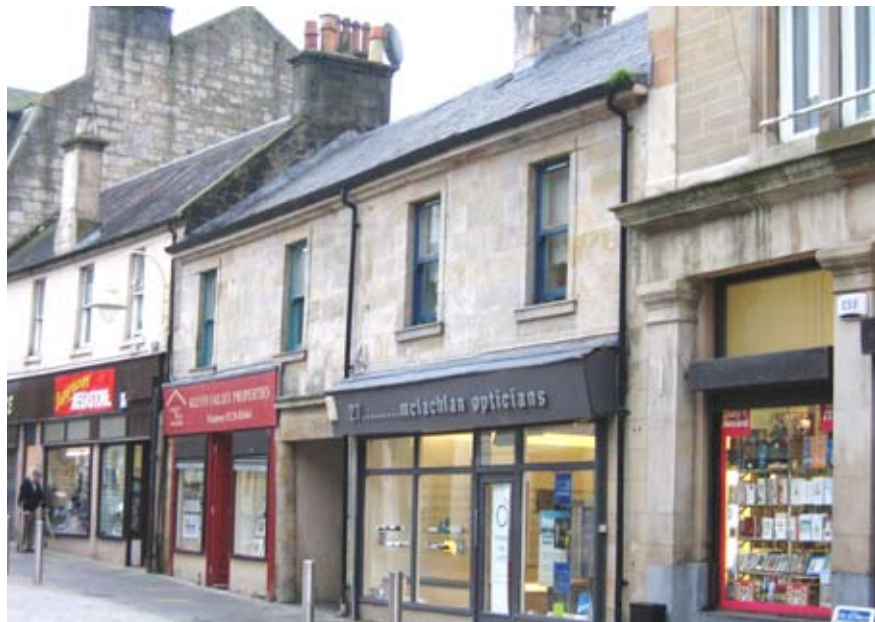
Shopfront design is a key element of successful retail areas. A well designed shopfront can have a positive effect on attracting and welcoming customers.
