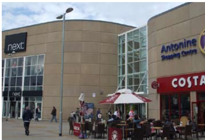
Modern signage should help identify the entrance and have some consistency - not simply use the wall as a display board
