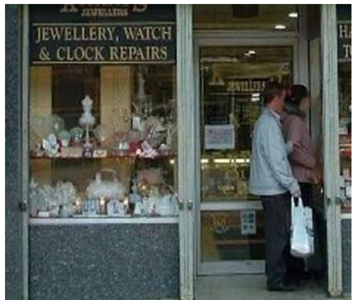
Reinforced stallriser providing additional security
