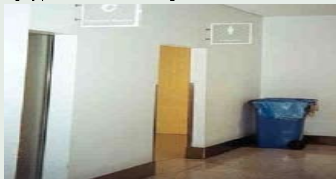
Poor colour contrast makes wayfinding difficult
