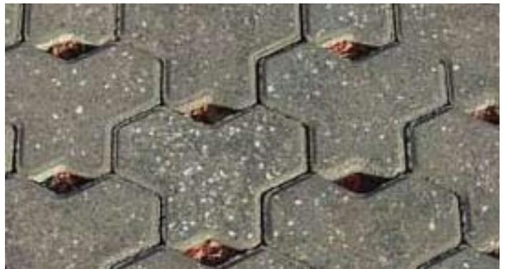
The use of porous paving and blocks can help rainwater drain away naturally saving significantly on underground pipework.
