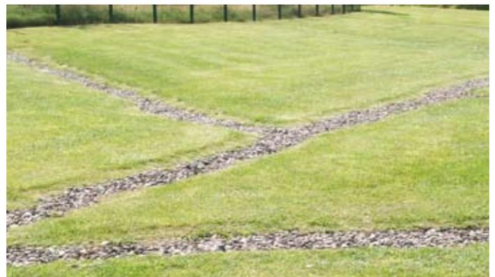
Example of Sustainable Urban Drainage - A filtration trench which slows and removes pollutants from run-off
