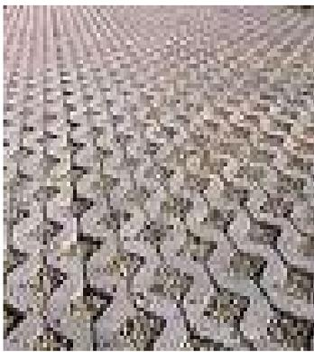
Purpose designed permeable paving slows runoff.
