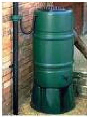
Water butts can aid flood prevention by source control
