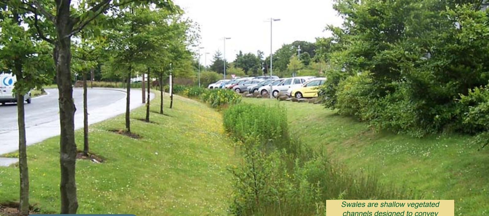
*Swales are shallow vegetated channels designed to convey road runoff and treat pollutants (from Scots "SUDS for Roads")*
