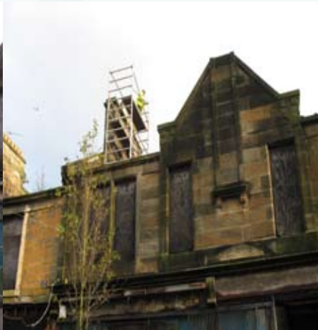
The Whitehouse Jan 08 during works undertaken through an Urgent Works Notice
