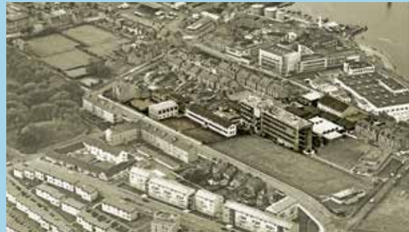
C BLOCK BEING BUILT
