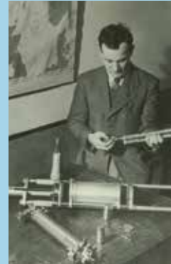
PARRISH PREPARING A NANSEN BOTTLE AND REVERSING THERMOMETER
