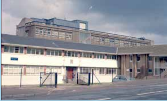
BLOCK A, PRIOR TO REFURBISHMENT
