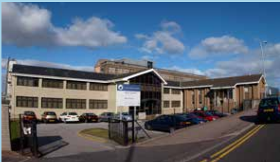
BLOCK A, REFURBISHED AND UPDATED
