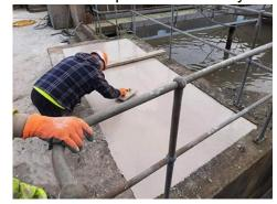
these is a product called 'Cemfree' - Cemfree can be used in place of cement to produce a low carbon concrete with up to 80% less embodied carbon.
