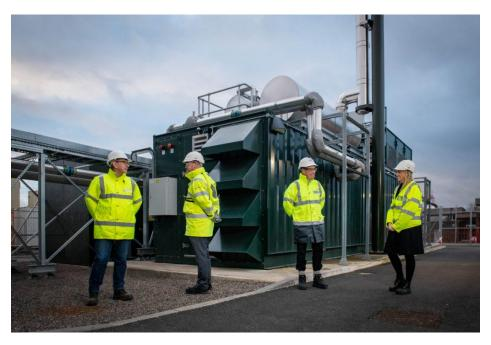
Built on-site at Scottish Water's Dalmarnock Waste Water Treatment Works, the system uses a mix of heat from waste water technology alongside a combined heat and power (CHP) engine to provide instant heat and hot water to homes and office buildings.
