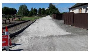
Traditionally, when repairing potholed roads, the existing road surface is dug up and replaced with aggregate which is made up of quarried sand, gravel and rock. Excavating and removing old materials and bringing in new materials (with associated use of transport and heavy plant) all add to the carbon emissions produced.
