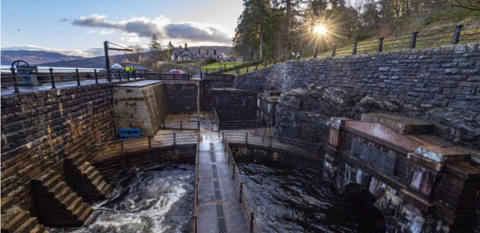
Picture 3 – Katrine Aqueduct
