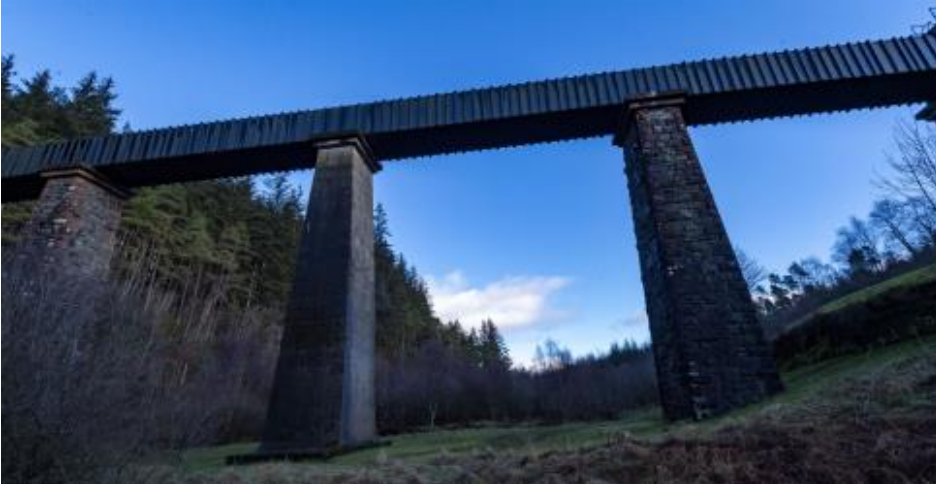
Picture 7 – Katrine Aqueduct
