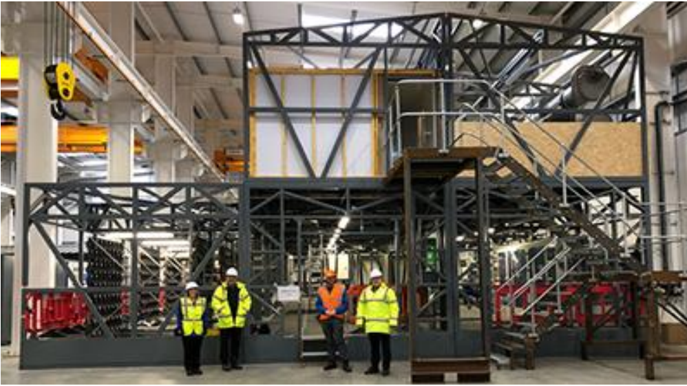
Picture 8 – Lochmaddy Water Treatment Works
