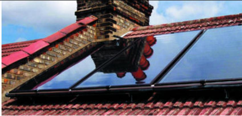
**Figure 5: Flat plate collector located above the roof covering** Source: Sabre systems
