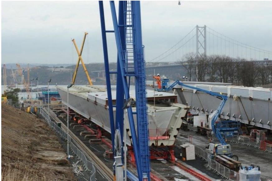
Construction of the Queensferry Crossing
