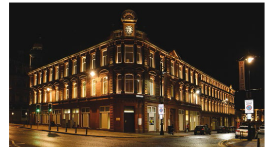
Civic Centre, John Dickie Street, Kilmarnock
