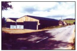
use a multi-span building rather than single span to reduce overall height and create a more varied roof line.
