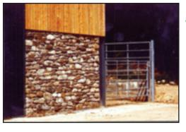
Consider the use of traditional materials to provide an important link with existing buildings. Treated timber is now an extremely versatile material with an extended life and, in particular, can be effectively used as space boarding where natural ventilation is required; and
