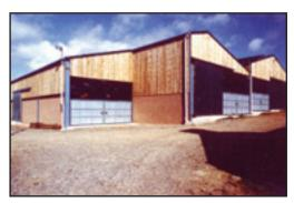
break up large expanses of roof and walls with well designed and carefully positioned functional elements such as roof ventilators, gutters, downpipes, doors and windows.
