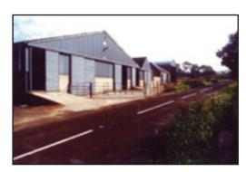
where possible match roof pitches with those on existing buildings. Although low pitched roofs can make a building less obtrusive, they are often out of harmony with the steeper pitches of older buildings. Steep pitches are also usually more appropriate within forest areas; and
