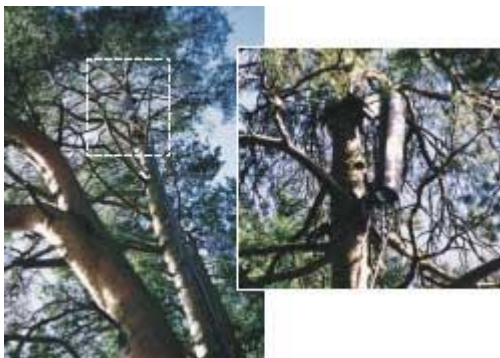
Directional antenna and feeder cable attached to a tree.
