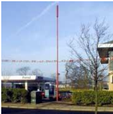
Monopole mast designed to fit the street scene.
