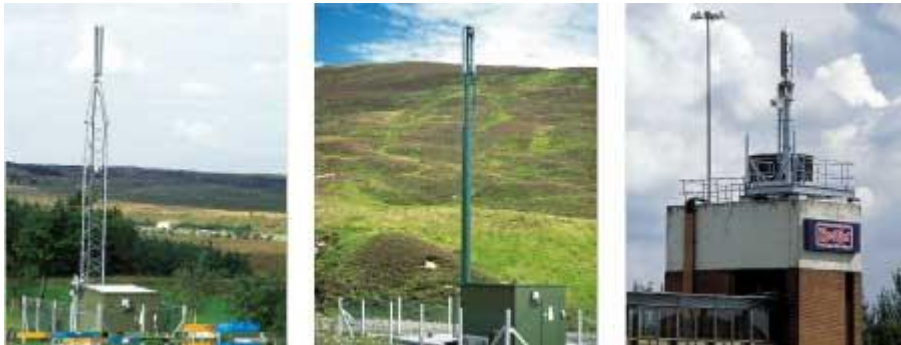
Second generation lattice mast, Second generation monopole mast and Second generation stub tower on rooftop.
