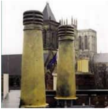
Equipment disguised as a chimney pot. Courtesy of The Undetectables.
