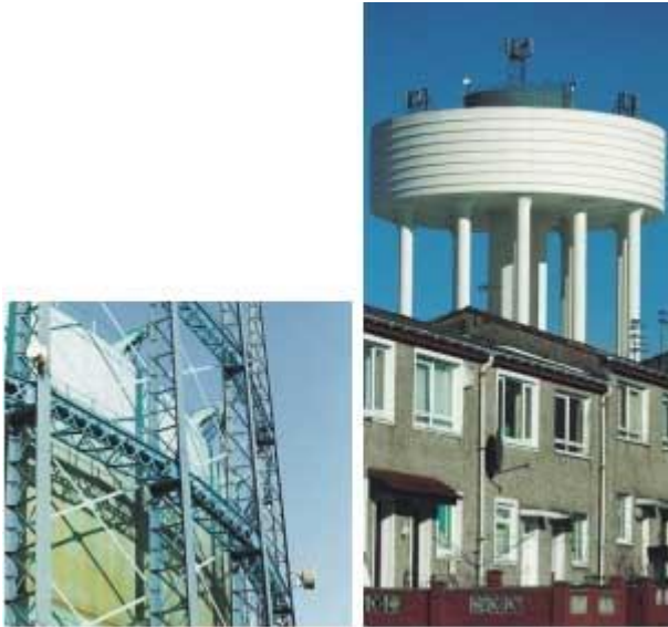
Siting equipment on a gasometer and water tower.
