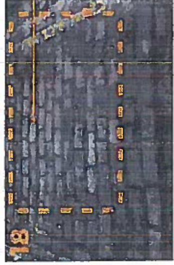
Natural stone setts appear to have been relaid within the past few years.
