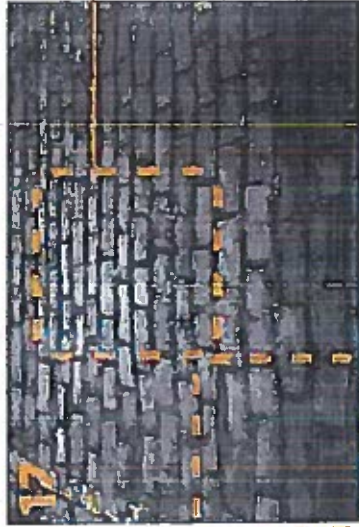
Setts appear to have been repaired and reinstated using a variety of bedding and jointing techniques.
